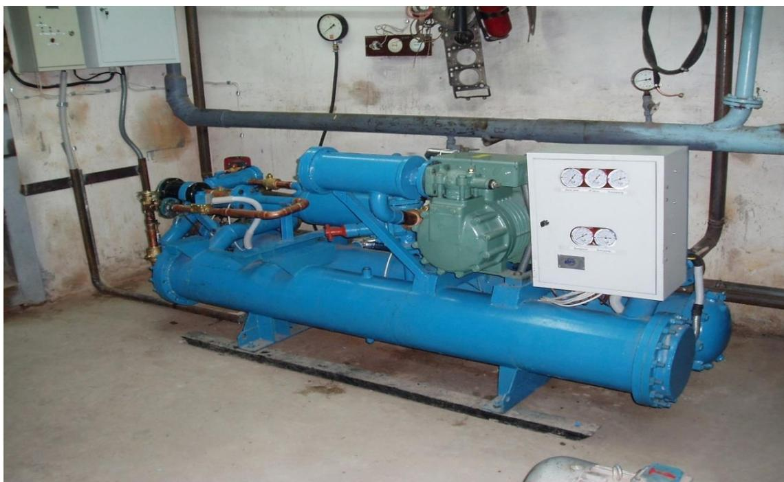
**Figure 2.** The HP NT-60-1 for the heat supply of the Baikal Museum of the Scientific Center of the Siberian Branch of the Russian Academy of Sciences on the basis of renewable heat of Lake Baikal water
