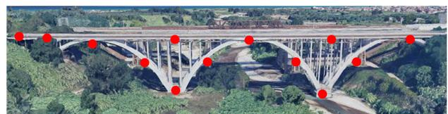
Fig.5 - Sensor positioning.
