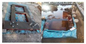
Fig.1Casting and curing of RC frame model
