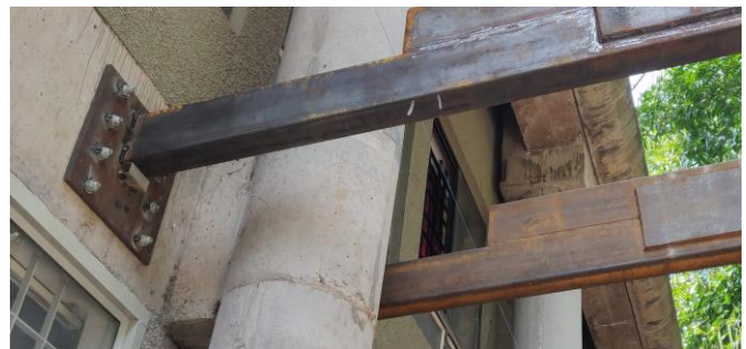
Fig. 1. a) Cantilever beams for structural support of an extended ceiling in the College Campus b) Joint mechanism.
