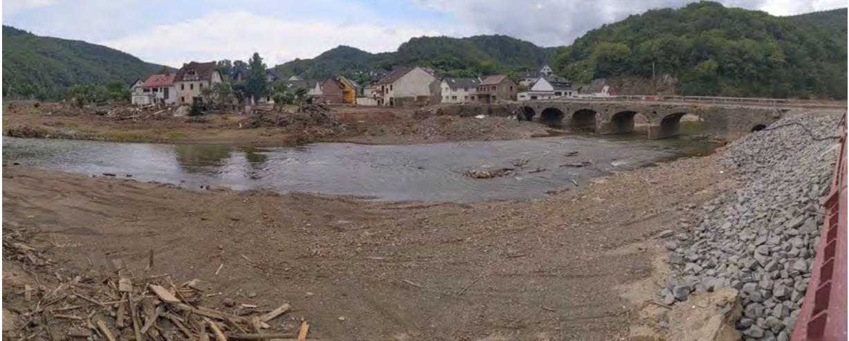
Figure 3.102. Ahr bridge Brück (road bridge) with temporary fill placed on the right arch to enable bridge passage (50.4866352, 6.9717177)
