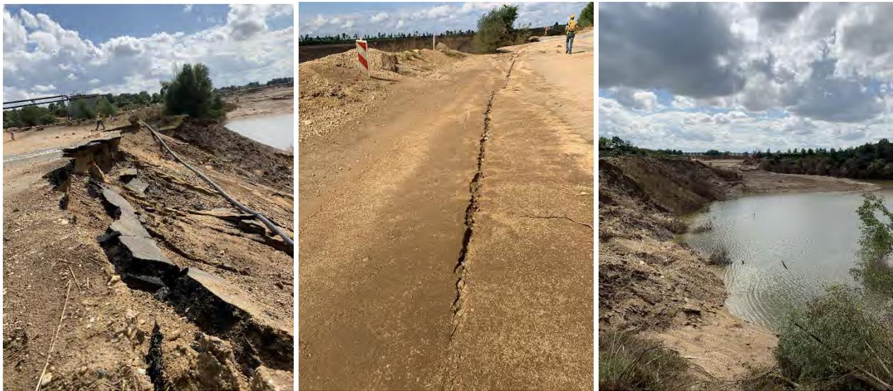
Figure 3.41. Left: Damage to asphalt gravel roads; Center: Soil cracks possibly indicated deeper seated slip surfaces; Right: Water levels of the gravel pit at the time of the team visit (50.818468, 6.794142).
