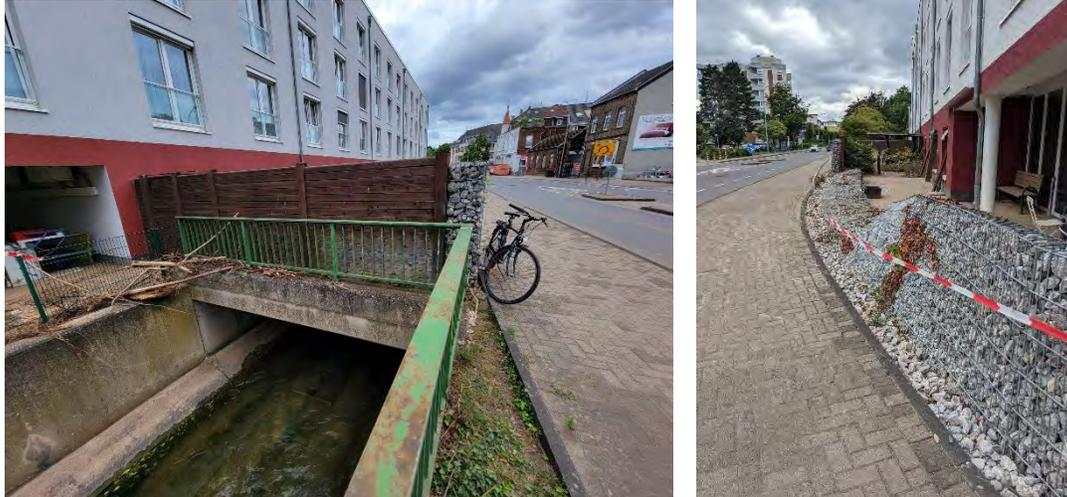
Figure 3.18. Bridge over small Erft tributary (Veybach) which obstructed the river flow (left), damaged gabion wall immediately behind the bridge (right), (50.6579006, 6.78616520)
