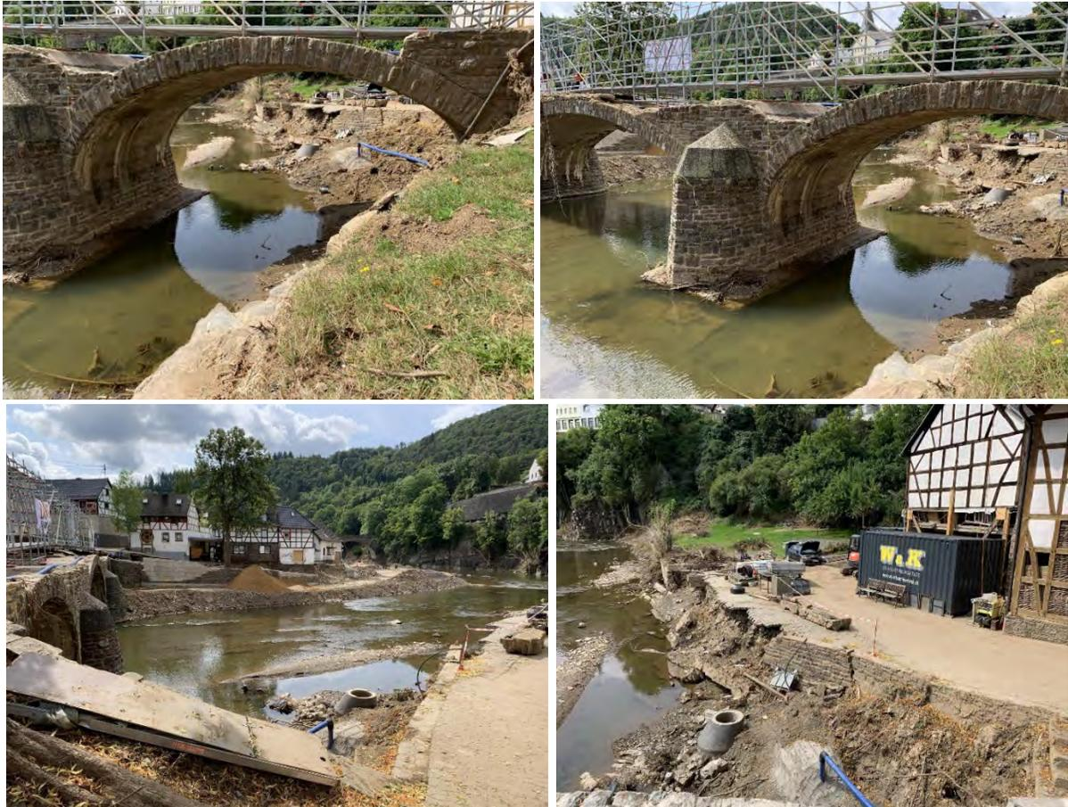
Figure 3.74. Top: damage around the bridge superstructure, bottom: massive amounts of riverbank erosion and the temporary fill (bottom left); (50.4481131, 6.8901355)
