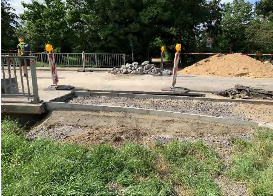
Figure 3.50. Erosion suggested flow from the road down the riverbank's slopes created damage to the pedestrian path of the bridge section connecting with the riverbanks (50.782199; 6.822505).
