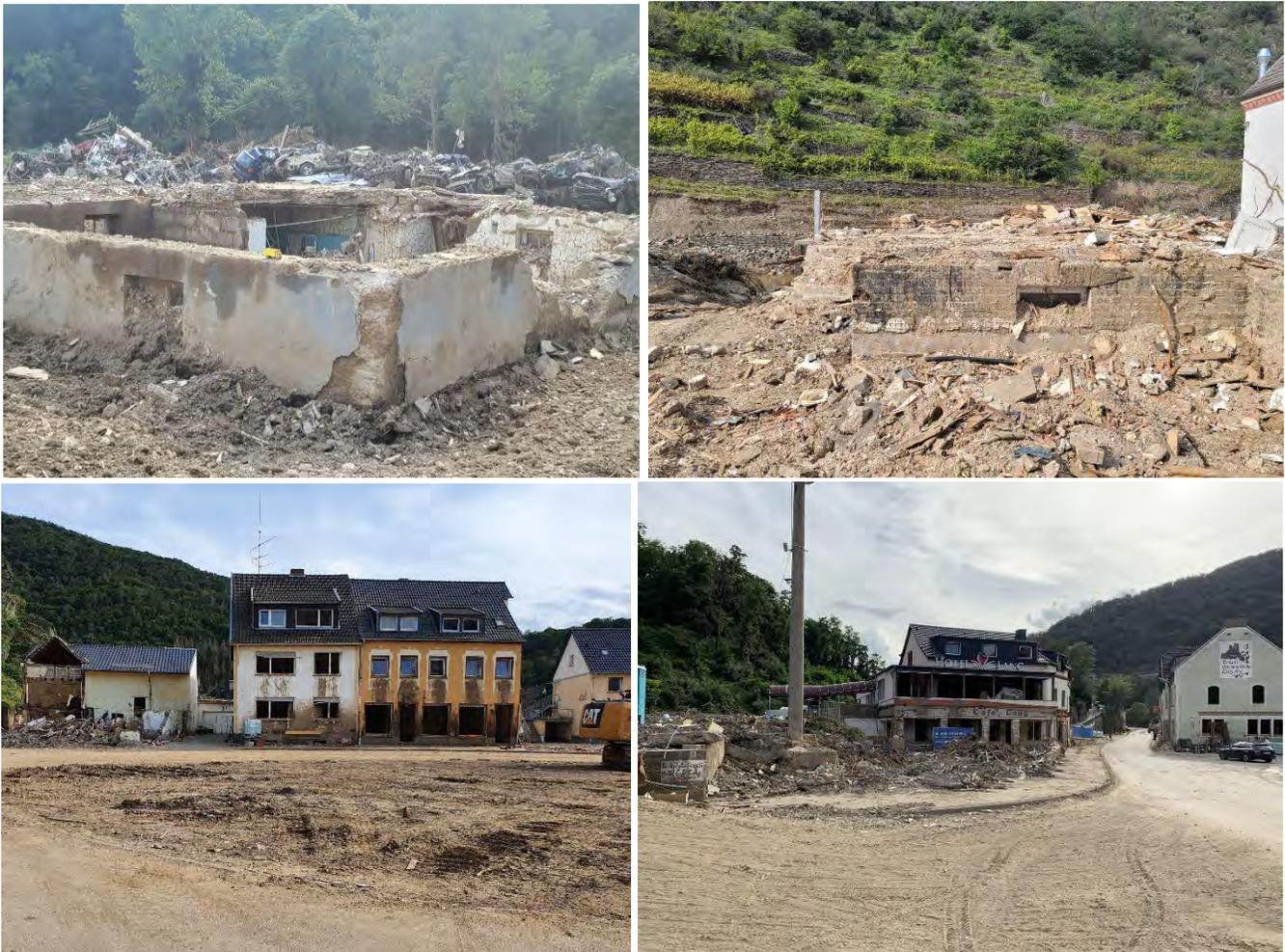
*Figure 3.145. Photos of damage and destruction in the town of Altenahr by the GEER team; top: houses destroyed to the foundation level, bottom: houses flooded until roof level (50.51671855, 6.9903993)*
