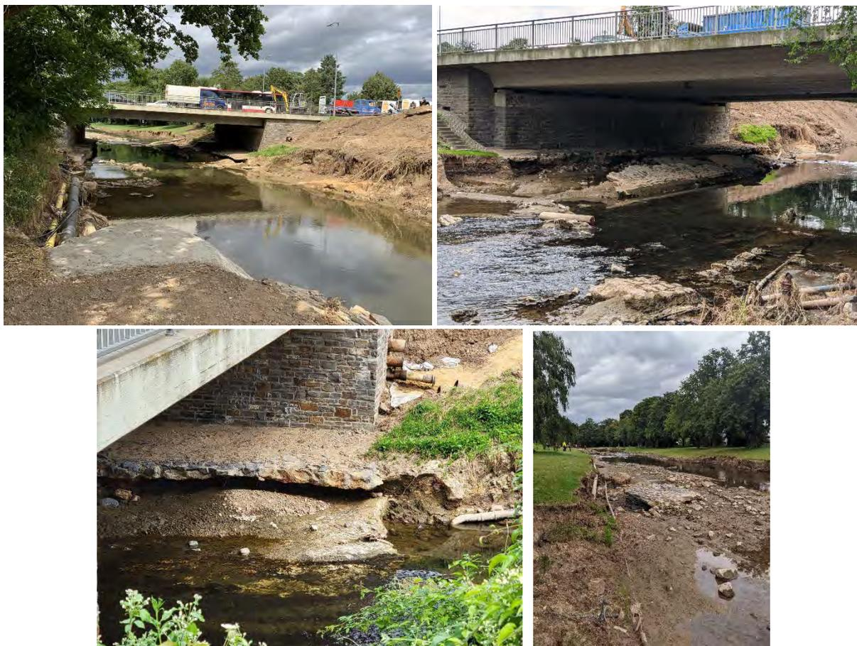
Figure 3.21. Scour damage at the foundation level of the Road bridge across the Erft @ Kölner Strasse (50.660347, 6.805227).
