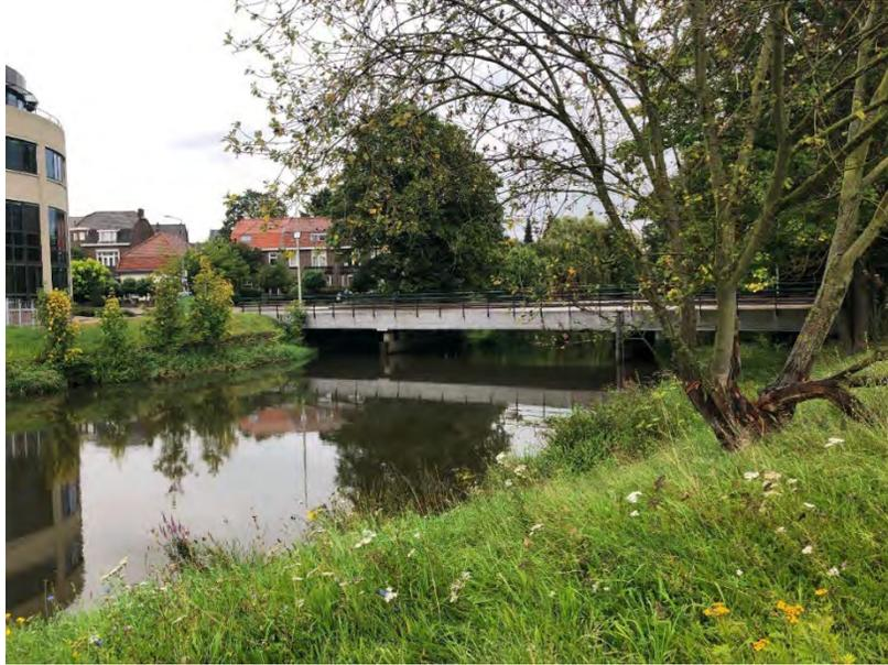
Figure 3.277. Approx. 50 meters from the intersection of the Roer and Hambeek rivers, a road bridge shows no signs of scour along the piers or embankment. Water levels did not breach the deck. (51°11'06.6"N 5°59'19.4"E)
