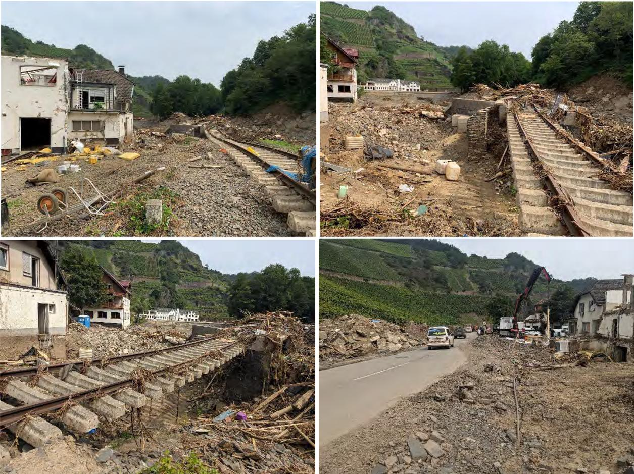
Figure 3.213. Damage documented around the rail bridge and adjacent residential building (50.532217, 7.0624500)
