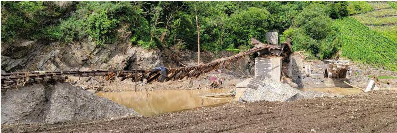
Figure 3.190. Panoramic view of destroyed rail bridge at Hotel Bergischer Hof. Photo Credit: Heinz Grates accessed through: [https://www.aw-wiki.de/index.php/Ahrtalbahn-Br%C3%BCcke\\_Mayscho%C3%9F](https://www.aw-wiki.de/index.php/Ahrtalbahn-Br%C3%BCcke_Mayscho%C3%9F)
