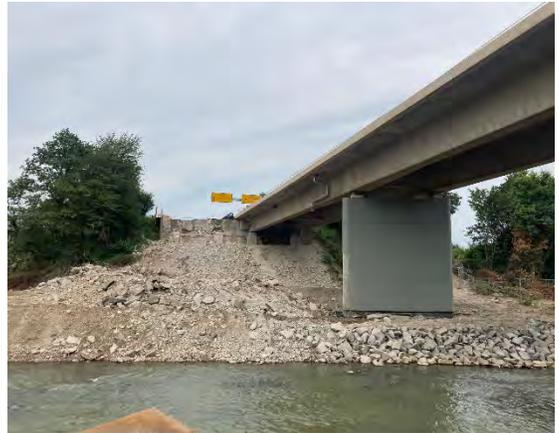
Figure 3.231. B9 bridge in Sinzig (left) shortly after the flood event, Source: [blick-aktuell.de](http://blick-aktuell.de);
