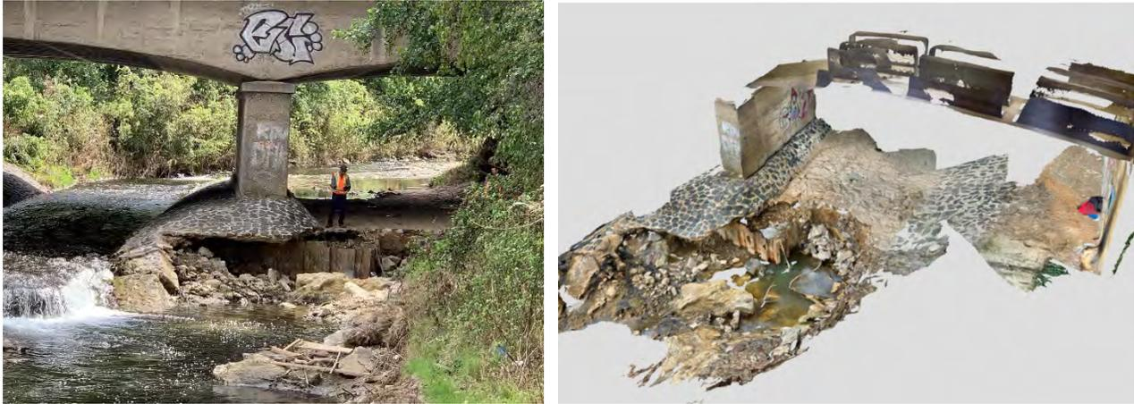
Figure 2.2. Photograph (left) and LiDAR model (taken with the iPad Pro 2020) (right) of scour damage at foundation level of railroad bridge crossing river Erft, parallel to Kölner Straße
