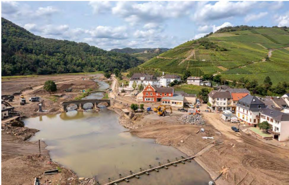
Figure 3.198. Rech and the destroyed Nepomuk bridge (middle) with a pedestrian emergency bridge (front) and two road bridges (background)
