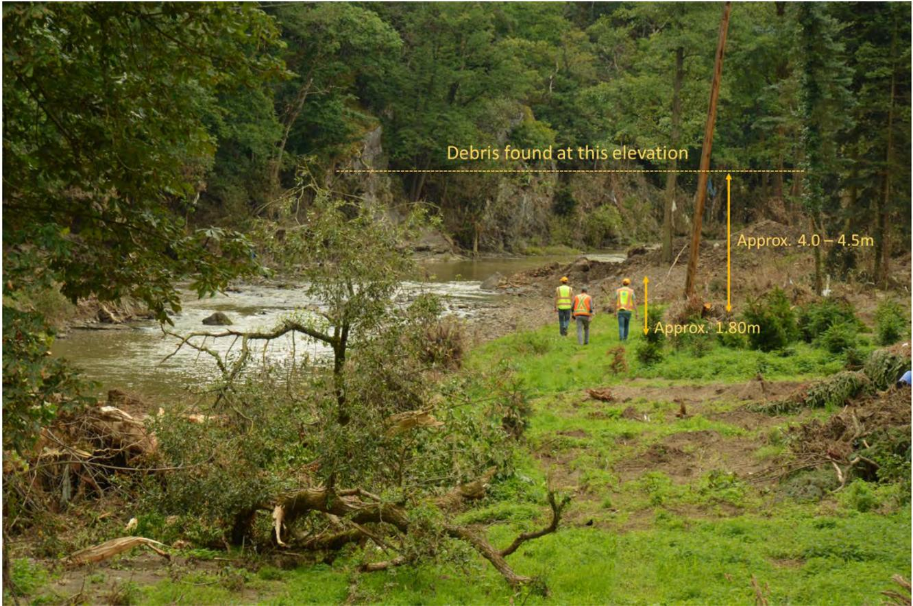
Figure 3.62. Team members walking upstream of the bridge inspecting damage and debris deposits along the riverbanks (50.43275924, 6.85851324)
