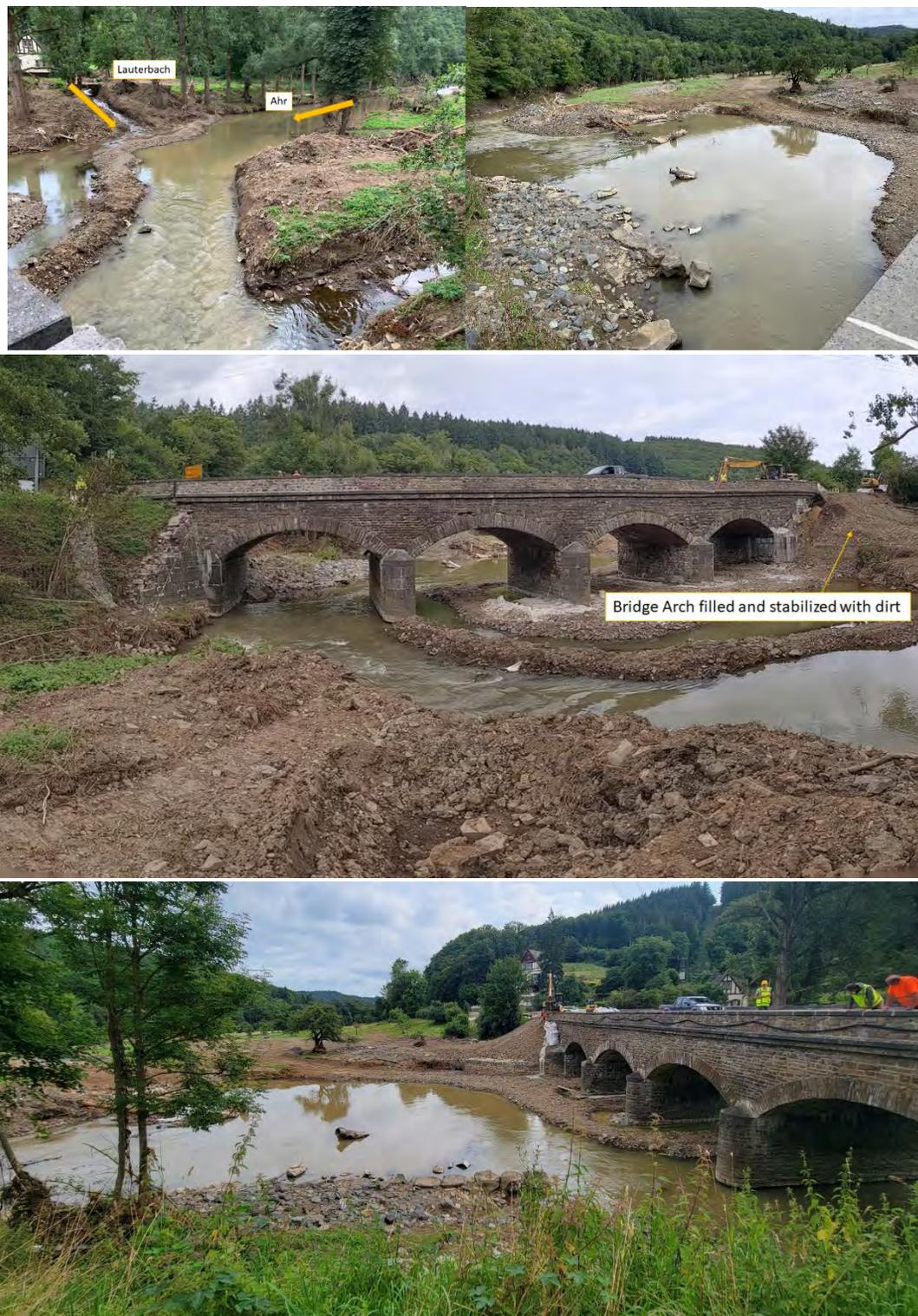
Figure 3.63. Upstream (top) and downstream (bottom) side of the bridge showing fill soil in lieu of bridge arch (50.432840, 6.858008)
