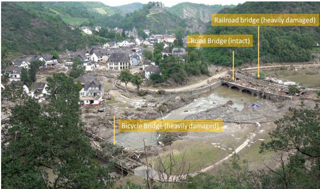
Figure 3.132. View of damaged bridges near campground Viktoria-Station, Altenahr (photo: picture alliance/dpa)
