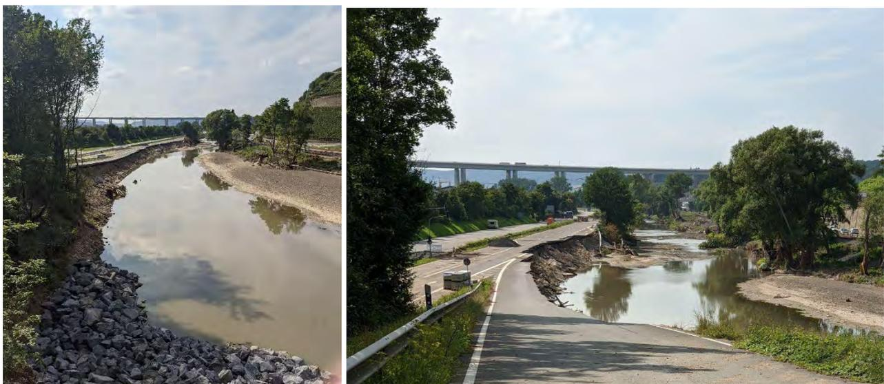
Figure 3.225. Shift of the Ahr river to adjacent to the B266 and associated road damage (50.5465709, 7.1828458).
