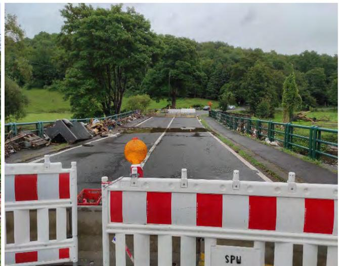
Figure 3.260. Damage to Louheau bridge which links Pepinster to Trooz via Nessonvaux on the N61 in Wallonia, Belgium. Excessive settlement of the middle pier foundation (top). Before flooding (source: google street, April 2021). Exact location 50°34'1.32"N, 5°46'56.
