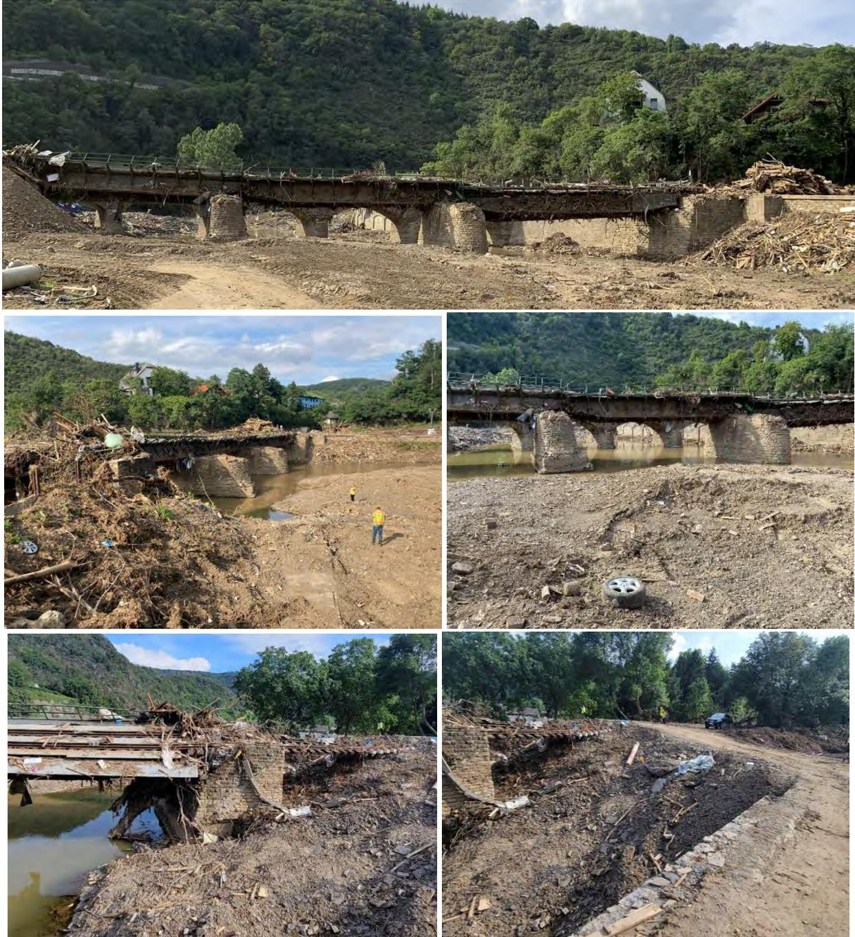
Figure 3.134. Photographs of the damaged rail bridge (top and center) and washed-out abutment region (bottom), (50.5147775, 6.98626321)
