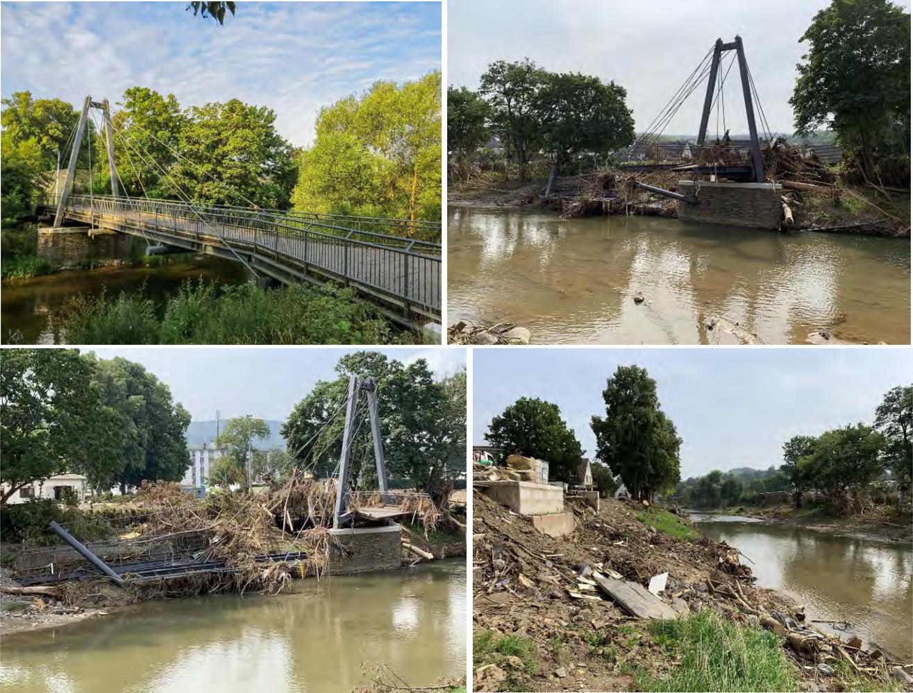
Figure 3.223. Otterbrücke, Bad Neuenahr Ahrweiler. top left) before the flood event top right & bottom left) destroyed bridge deck, rotated counterclockwise in downstream direction on August 12, 2021; bottom right) bridge abutment (downstream left), structurally intact at the time of the team's visit (50.53874, 7.1013125)
