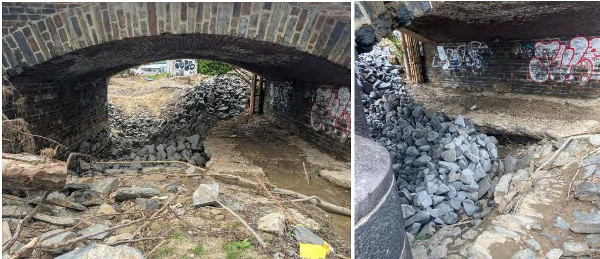
Figure 3.229. Infill of the scour hole and of an erosion channel suggesting flow from the top of the upstream northern riverbank down through the northernmost bridge arch (50.549856, 7.244673).
