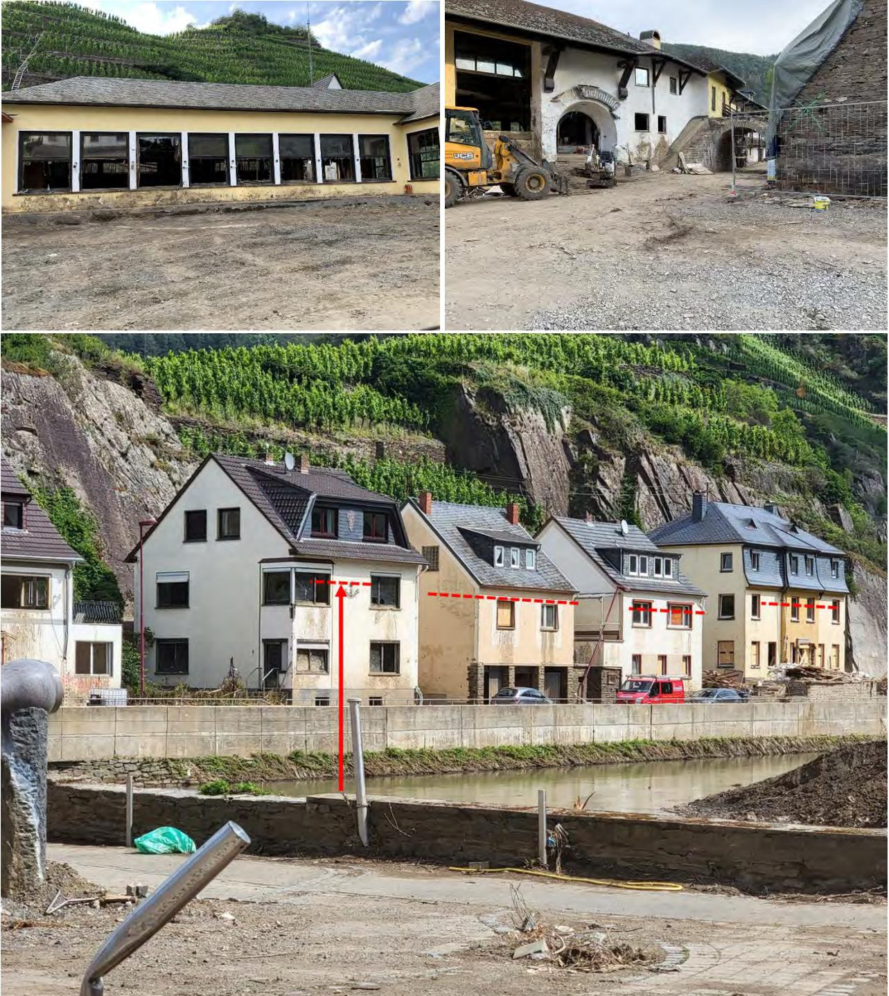
Figure 3.181. Top: Remains of a flooded winery in Mayschoss; Bottom: watermarks at several residential buildings along Bundesstrasse 267 in Mayschoss indicating water level rise during flood (50.52194645, 7.021036269)
