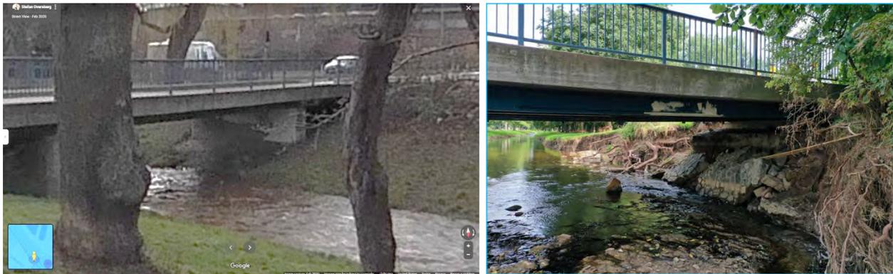
Figure 3.25. Bridge Crossing before flood per Google maps (left), Bridge after flood at time of teams visit (right). (50.6668240, 6.7988197)
