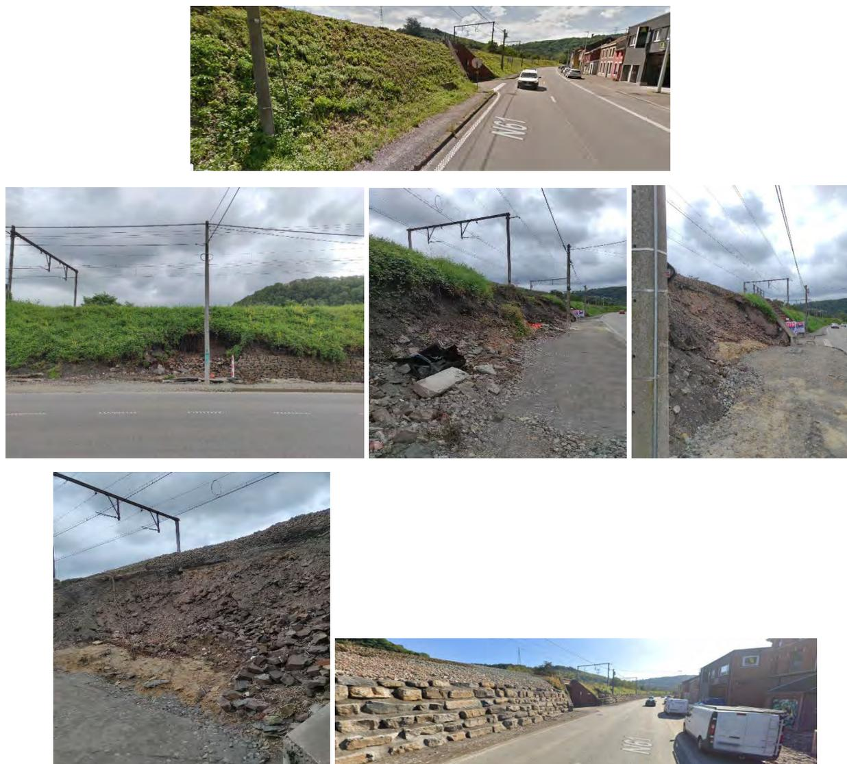
Figure 3.246. Embankment failure along railway 37 near Chaudfontaine (50° 35' 51.58" N, 5° 37' 53.38" E); top: before the flooding (June 2019, Source Google street view), Center and Bottom left: Failure documented by the GEER team, Bottom right: after repair works (October 2021, source google street view)
