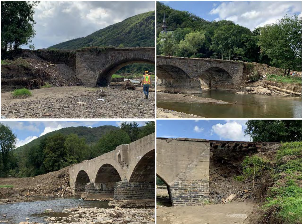
Figure 3.117. Damage and Erosion around the bridge abutments. From downstream direction (Top left and right) and upstream direction (Bottom left and right abutment), (50.4943691, 6.9822398).
