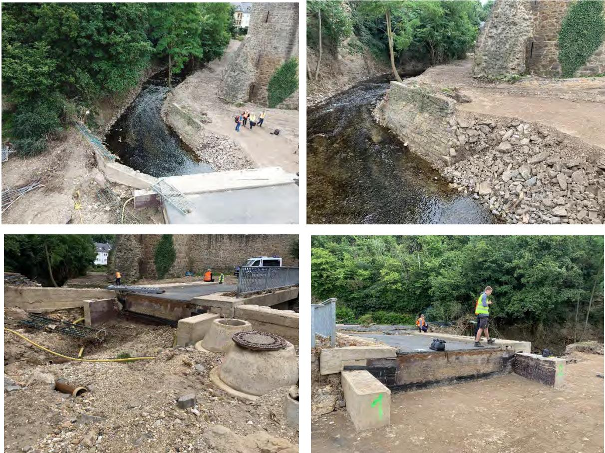
Figure 3.11. Damage around the bridge, riverbank damage (top row), bridge on-ramp and off ramp damage with severely scoured surface material and exposed manholes (50.557325, 6.7658949)
