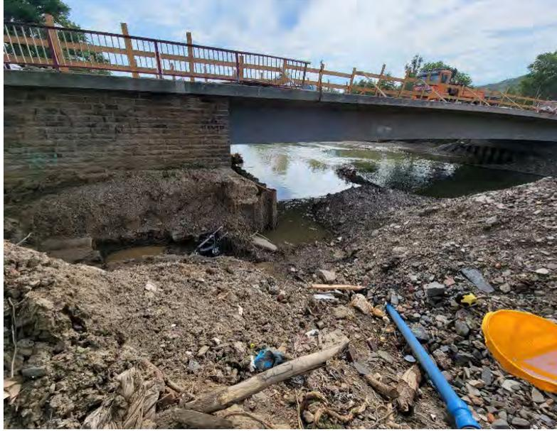
*Figure 3.222. Close up of the St. Pius Bridge pier in Bad Neuenahr-Ahrweiler separating the pedestrian underpass part of the bridge from the river crossing span. Significant scour is observed wrapping around the upstream part of the pier (50.542423, 7.115540328).*
