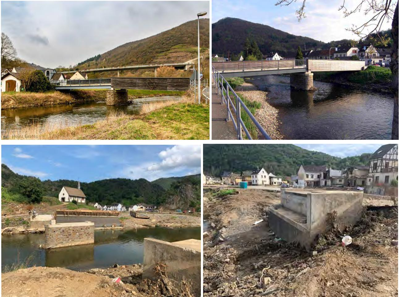
Figure 3.126. Top: Road bridge in Altenburg before flood (Source: <https://www.aw-wiki.de/w/index.php?curid=40670>) After: Bridge damage in Altenburg (GPS: 50.511551, 6.985069)
