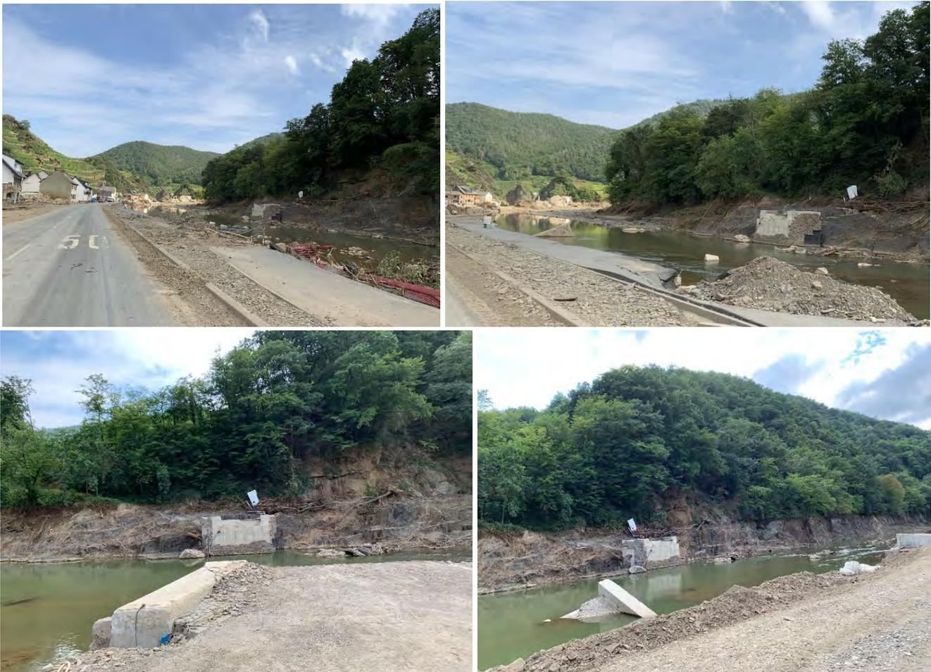
Figure 3.176. Remaining abutment structures of the pedestrian timber bridge Laach at the time of the team's visit (50.517824, 7.00952)
