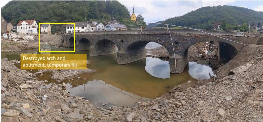
Figure 3.104. Bridge and temporary retrofit to missing arch and superstructure (50.4866352, 6.9717177).
