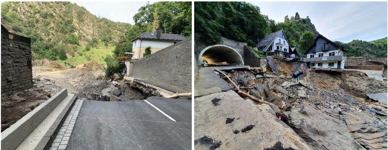
Figure 3.158. Cut-off of Tunnelstrasse at the Altenahr tunnel exit. View from inside the tunnel (left) and immediately outside the tunnel (right), (50.51631664, 6.9968335).
