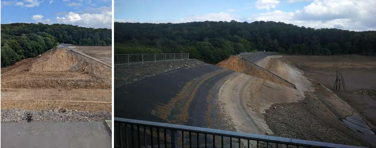
Figure 3.53. Left: Open cross-section of the Steinbachtalsperre during the team visit when repair was ongoing. Right: Reservoir-side view of the removed center part of the dam (50.594124; 6.838211).
