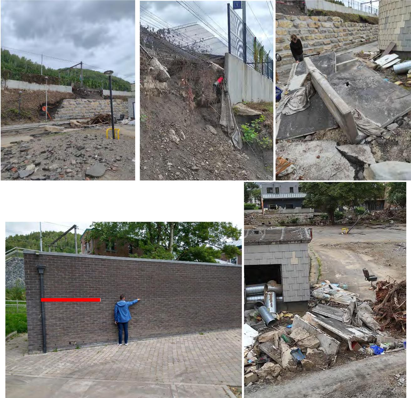
Figure 3.249. Railway embankment failure at Chaudfontaine Railway station; indication of water level during the flooding (exact location 50° 35' 13.02" N, 5° 38' 29.67" E)
