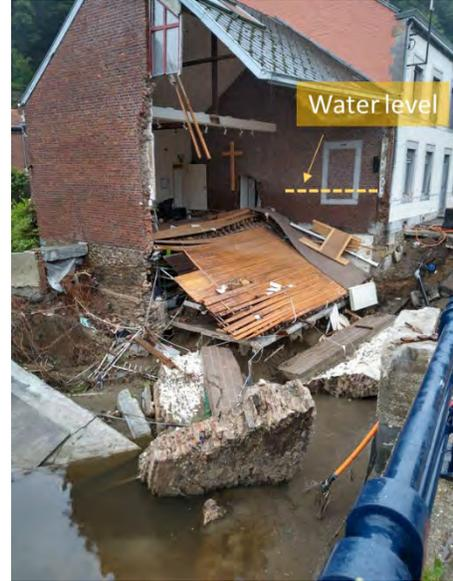
Figure 3.255. Photographs before (left - google maps) and after (right) damages in the Centre Protestant de Nessonvaux near a Vesdre river bridge abutment in Nessonvaux (50.574176, 5.742544)
