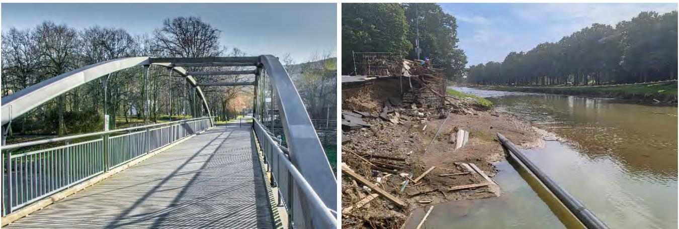
Figure 3.219. Left: Amseltal bridge before the flood event (source: [https://www.aw-wiki.de/index.php/Ahrbr%C3%BCcken\\_im\\_Kreis\\_Ahrweiler](https://www.aw-wiki.de/index.php/Ahrbr%C3%BCcken_im_Kreis_Ahrweiler)); right: Destroyed Amseltal bridge at the time of the GEER visit (50.542624927, 7.124041563).
