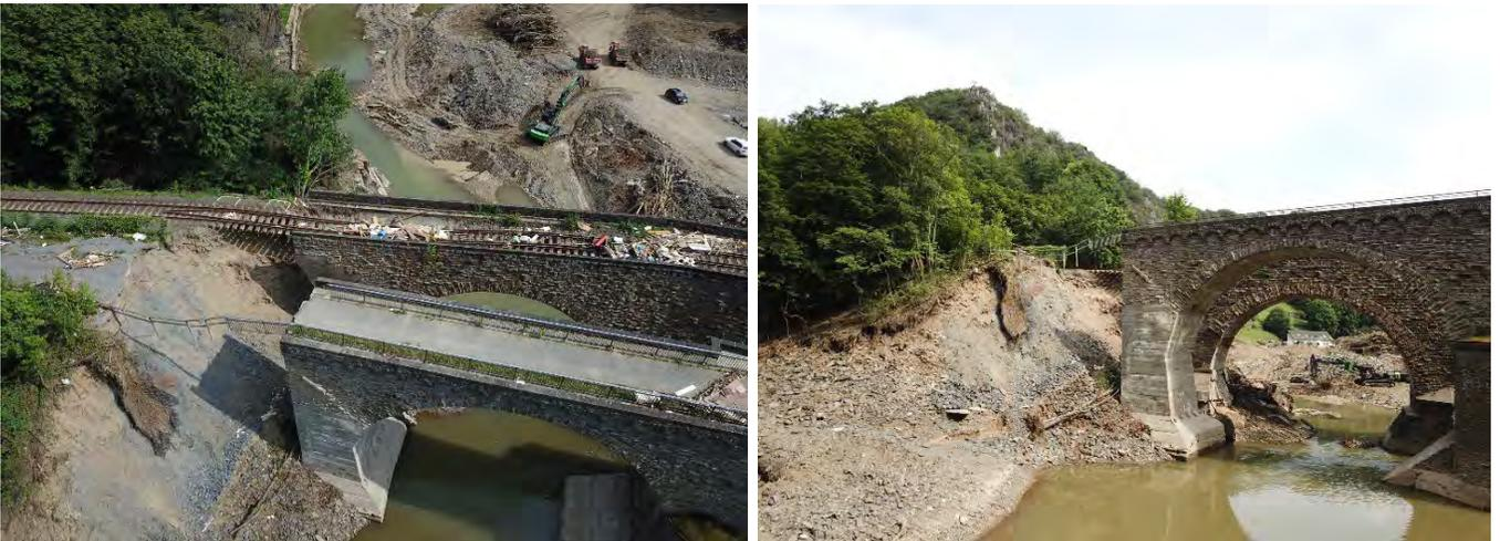
Figure 3.165. Major erosion around bridge abutment areas (50.5169260, 6.9970019).
