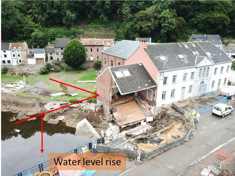
Figure 3.257. Aerial view of Centre Protestant de Nessonvaux and bridge abutment damage. Wingwall structural damage and soil erosion (top). Evidence of high-water level during the event (bottom), (50.574176, 5.742544).
