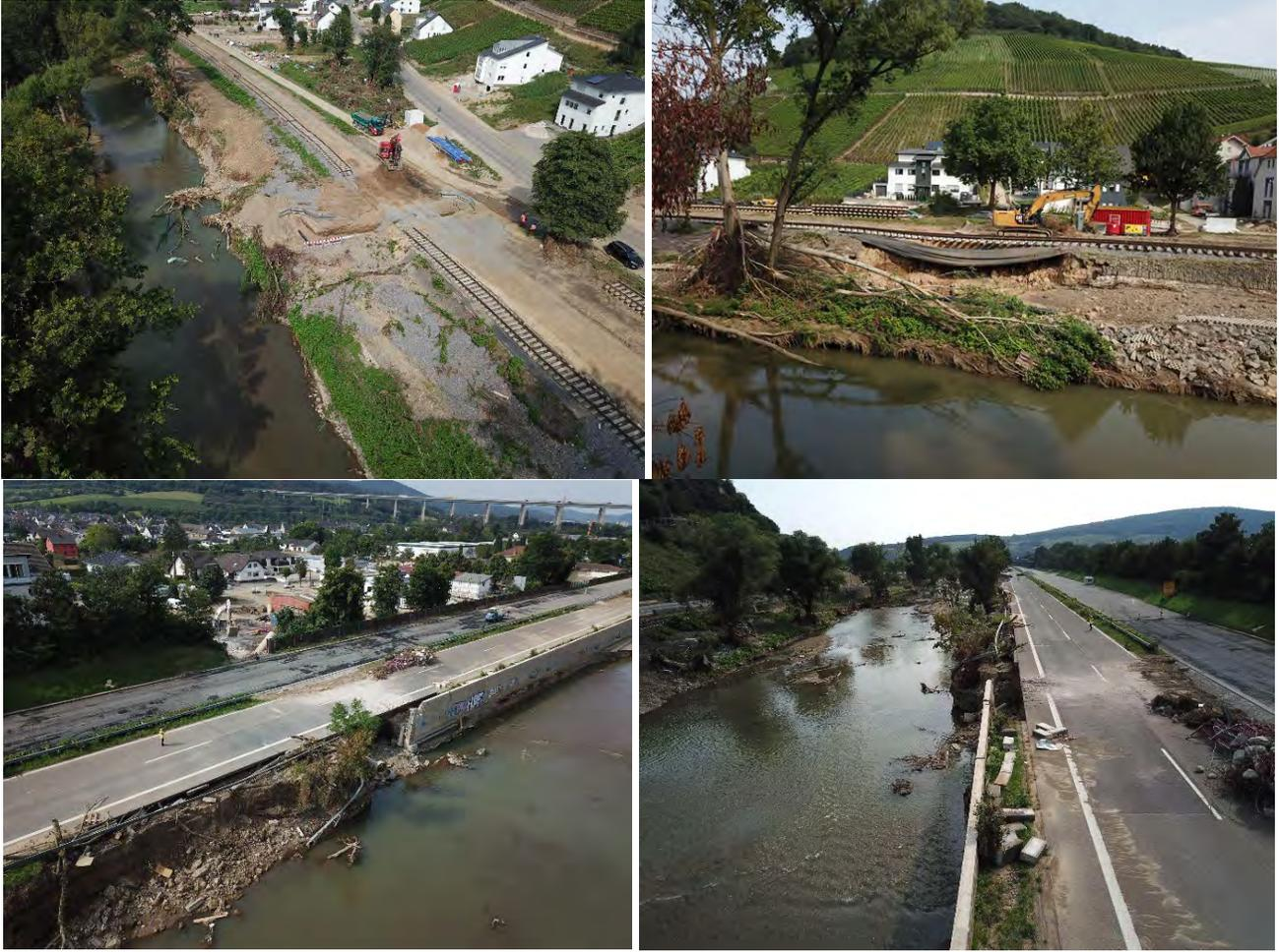
Figure 3.226. Rail damage (top) and embankment wall damage (bottom) along both sides of the Ahr river (50.547131515, 7.176075868).
