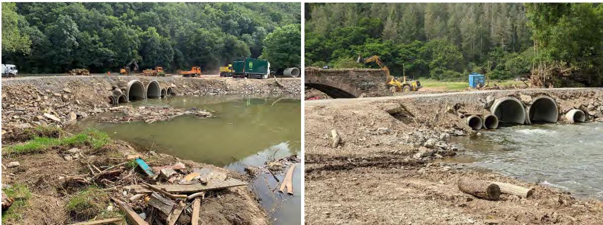
Figure 3.99. Concrete pipes and fill-based dam structure for temporary river crossing constructed by the Germany military; pipe inlet from upstream (left) and downstream (right) direction, (50.480833, 6.968818).
