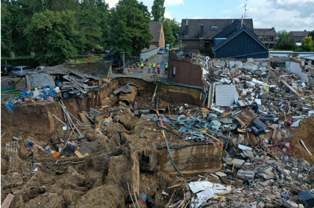
Figure 3.37. UAV image of the reconnaissance team standing at the edge of the Radmacherstrasse, exposed utility networks underneath the street (50.813582, 6.7950140).
