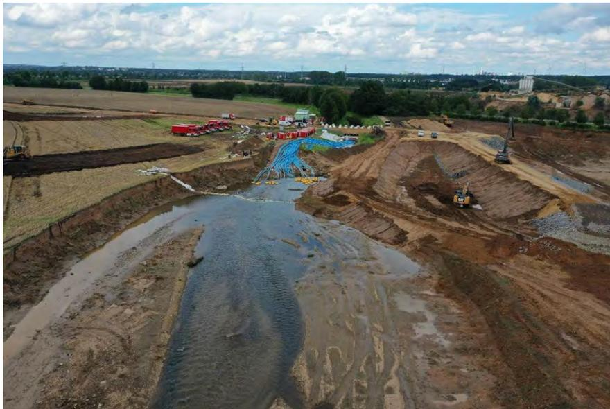
Figure 3.47. Aerial view of temporary dam and river rerouting by the Blessem fire department (50.8134771, 6.7890135).
