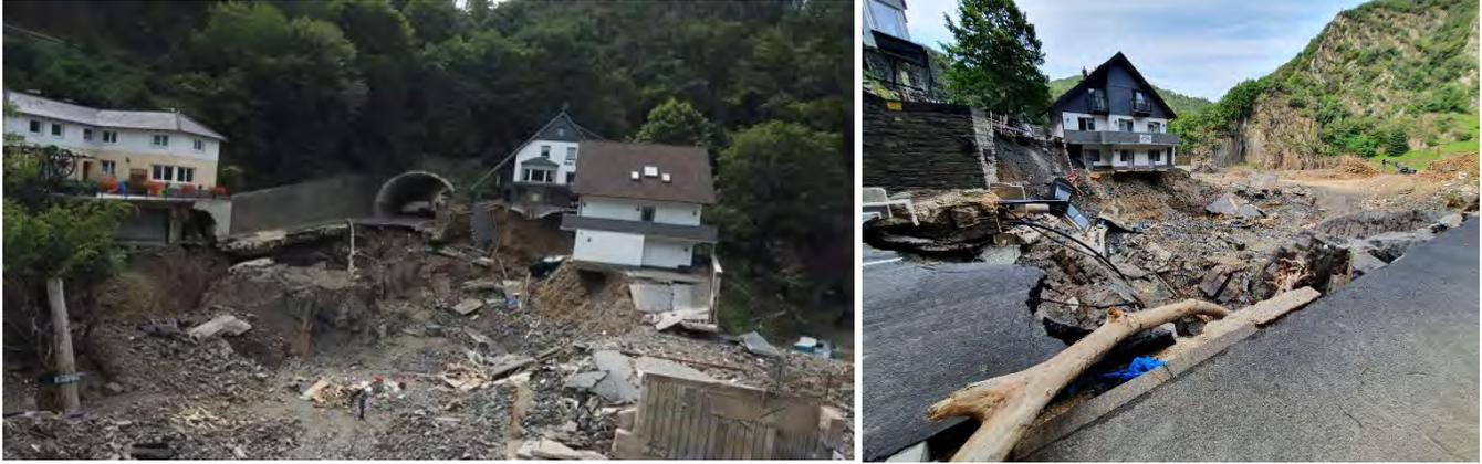
Figure 3.156. Destroyed Tunnelstrasse @ the tunnel exit following the 2021 flood (50.51631664, 6.9968335)
