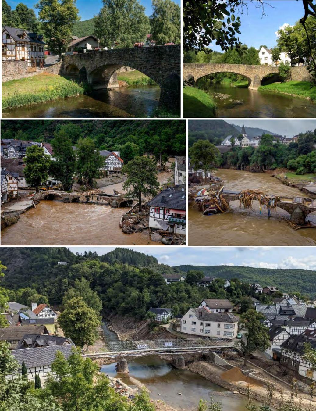
Figure 3.73. Top: Bridge along Domhofstrasse prior to the flood. (Fotos by Heinz Grates, source:<https://www.aw-wiki.de/w/index.php?curid=35184>), Center: Bridge at Domhofstrasse immediately following the flood, source: CNN on Facebook, Bottom: Bridge at Domhofstrasse on August 11<sup>th</sup>, 2021 at the time of the team visit., (50.4481131, 6.8901355)
