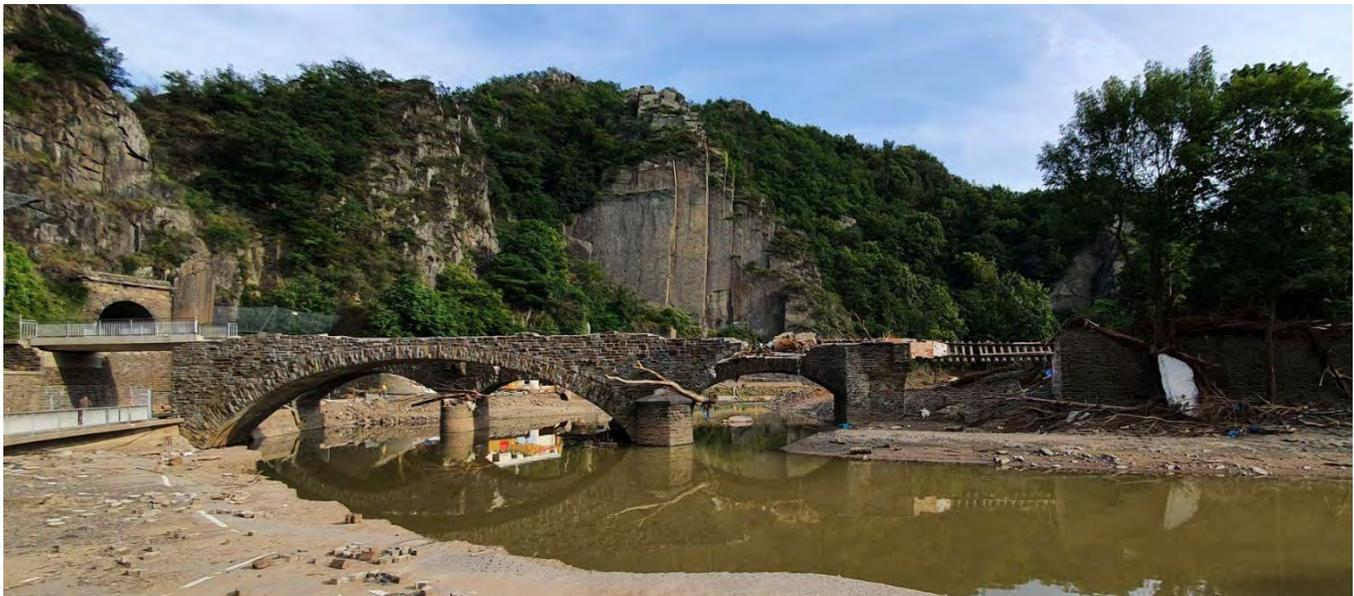
Figure 3.150. Photograph of remainder of the pedestrian bridge at tunnel entrance (front) and the severely damaged rail bridge in the back (50.5164851, 6.99482486)
