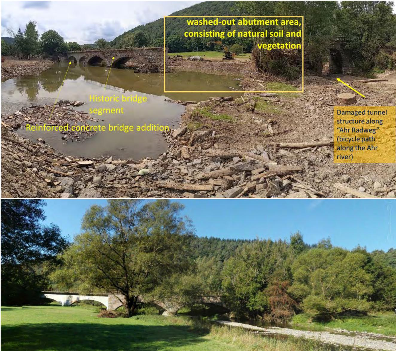
Figure 3.96. Comparison of post flood condition of the bridge and its surroundings (top, 50.480833, 6.968818) with pre-flood imagery obtained from google earth (bottom)
