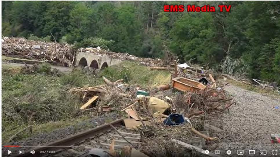
Figure 3.116. Railroad bridge shortly after the flood showing massive amounts of debris and deadwood piled up around bridge structure, Source: <https://www.youtube.com/watch?v=MSrJRXI6dQA>
