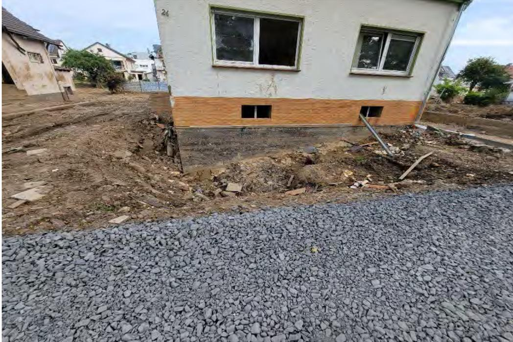
Figure 3.216. Residential building in Bad Neuenahr-Ahrweiler about 100 m from the Ahr river showing scour at corner of the building, destruction of yards and roads, and the original road just being temporarily replaced by a gravel road.
