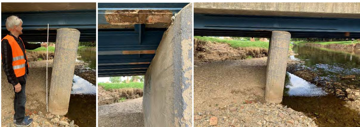
Figure 3.27. Shifted and tilted bridge pier with team member J. Stamm for reference (left). Horizontal movement of pier at deck interface (center), tilted support pier (right). (50.6668317, 6.7989968)
