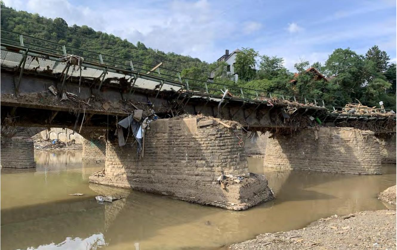
*Figure 3.135. Rail bridge: damage to bridge deck and tilted pier wall foundation(50.5147775, 6.98626321).*
