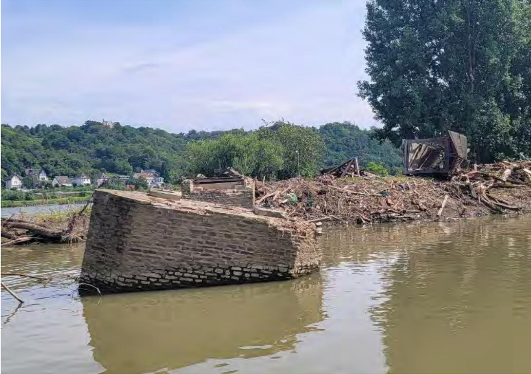
*Figure 3.236. Tilted bridge pier of Ahr-Rhine confluence bicycle bridge (50.558957; 7.276552).*
