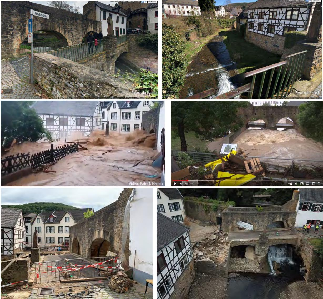
Figure 3.6. Picture of the Werkbruecke: Top row: Before flood (Source: google earth); Center: during flood (center) Source: Patrick Hamm one day after flood (July 16th), Source: [https://www.youtube.com/watch?v=7mZDH\\_P\\_1q4](https://www.youtube.com/watch?v=7mZDH_P_1q4) , Bottom photos: at time of teams visit, August 9th, 2021
