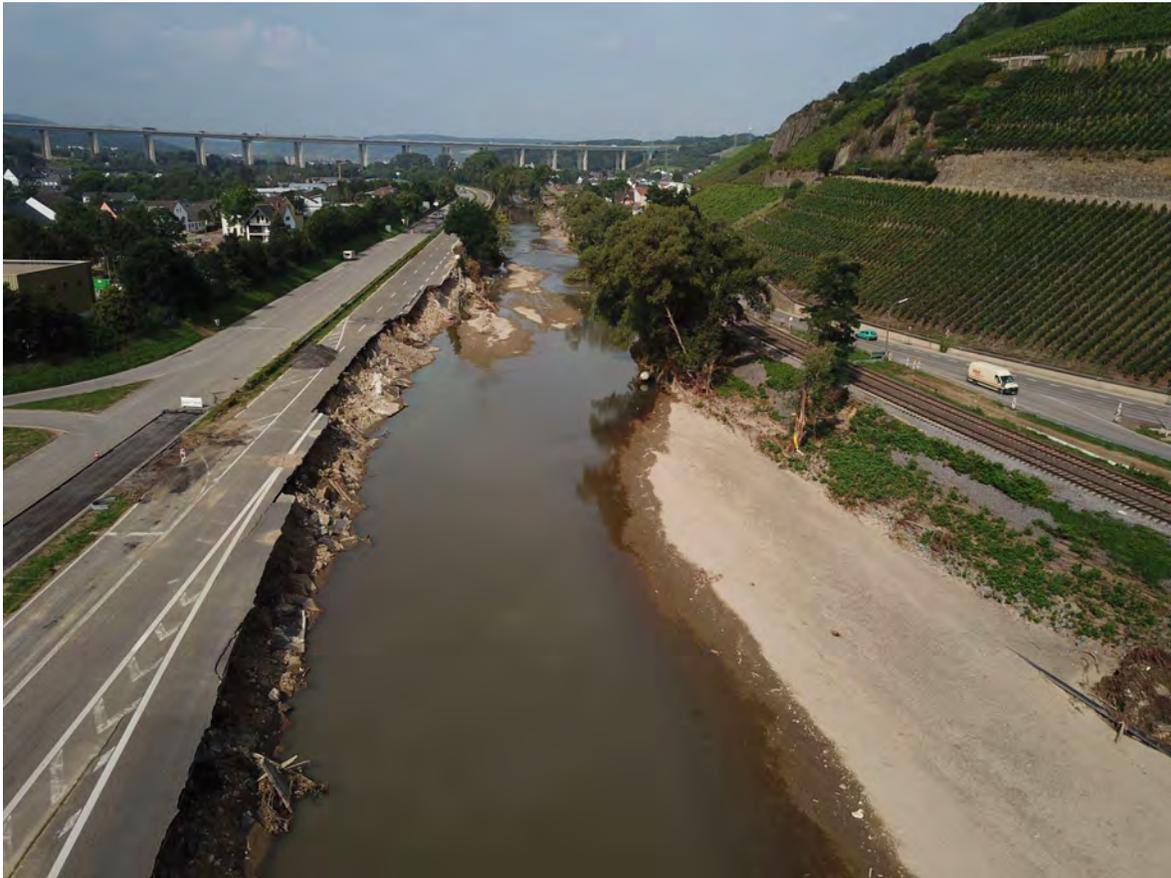
Figure 3.224. Overview image showing the Ahr river, undermining of B266 (left) and the railway tracks on August 12, 2021, after the flood (50.5468469, 7.1817397).
