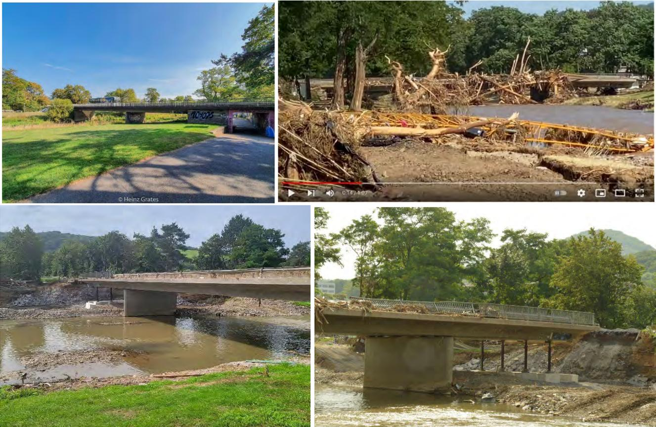
Figure 3.220. L83 bridge Bad Neuenahr-Ahrweiler. Top left: prior to the flood event (source: [https://www.aw-wiki.de/index.php/Ahrbr%C3%BCcken\\_im\\_Kreis\\_Ahrweiler](https://www.aw-wiki.de/index.php/Ahrbr%C3%BCcken_im_Kreis_Ahrweiler)); top right: significant deposition and accumulation of debris against and around the bridge during and shortly after the flood; bottom): the bridge at the time of the GEER team visit (50.542527; 7.121371)
