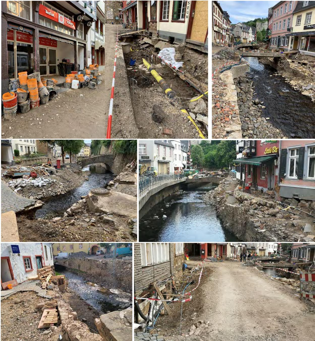
Figure 3.5. Damage to embankments, bridges, utility lines along the Ertf in the historic center of Bad Münstereifel (all photos by the GEER team)
