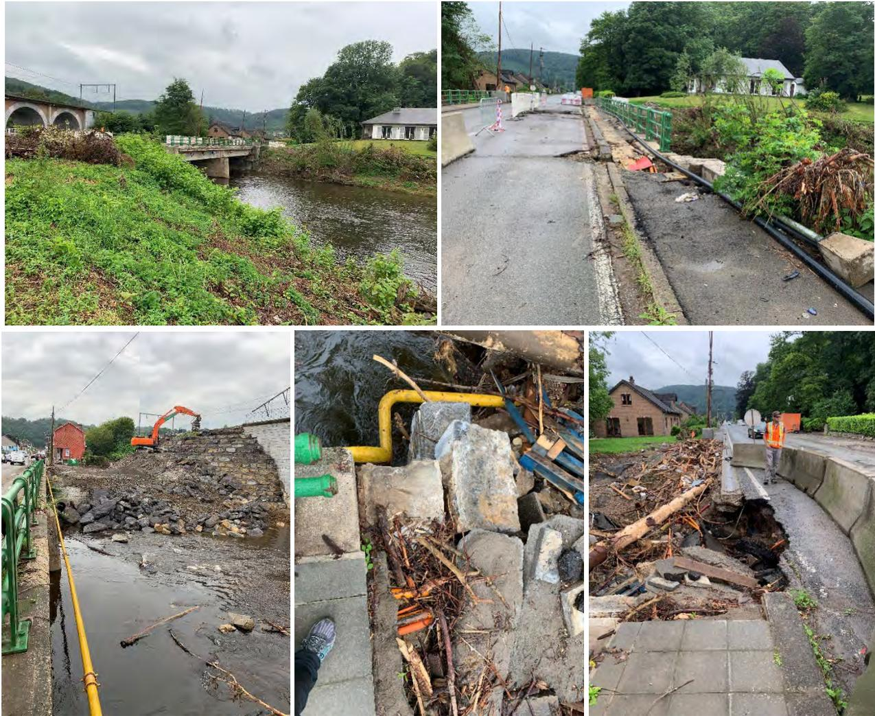
Figure 3.254. Damage of the road bridge along Rue Franklin Roosevelt (50°34'12.3"N, 5°44'13.7"E)
