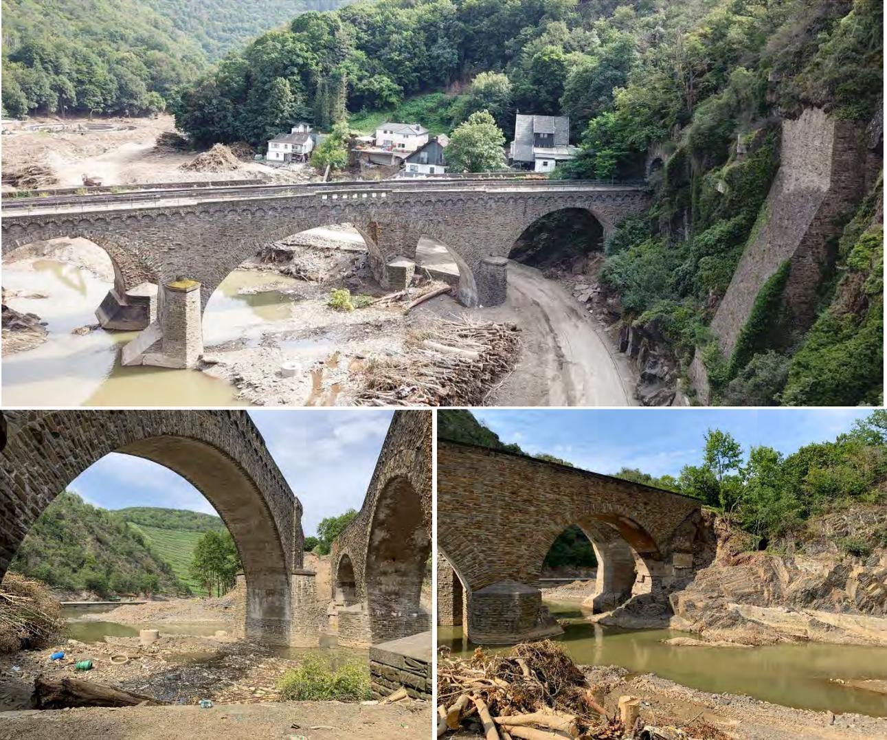
*Figure 3.166. Photographs of “double bridge”, showing mud fields and tree clean-up work (top photo) as well as erosion around bridge abutment and along the riverbanks (bottom photos), (50.5169260, 6.9970019).*
