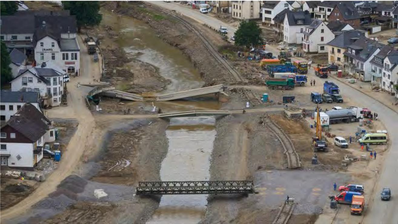
Figure 3.202. Damaged bridge with 2 emergency bridges (Jan 2022), Source: SWR.de, accessed through: <https://www.swr.de/swraktuell/rheinland-pfalz/koblenz/dernau-nach-dem-hochwasser-100.html>
