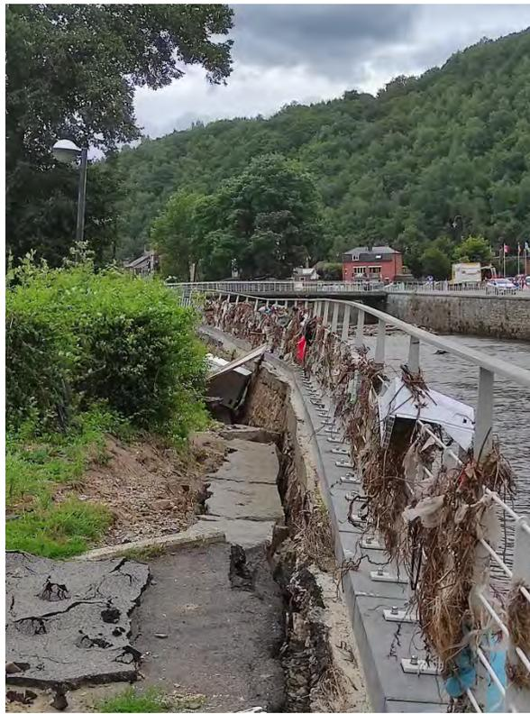
Figure 3.248. Embankment damage along the river near Chaudfontaine center (50° 35' 10.71" N, 5° 38' 34.46" E)
