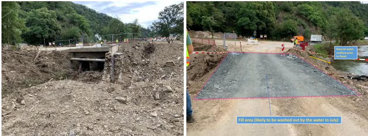
Figure 3.66. Bridge structure with 2 inlet arches (left), and destruction of surrounding areas; Dirt fill to re-establish road across bridge where waters have eroded the road and slope into the Ahr (right) (50.4470071, 6.8753387)
