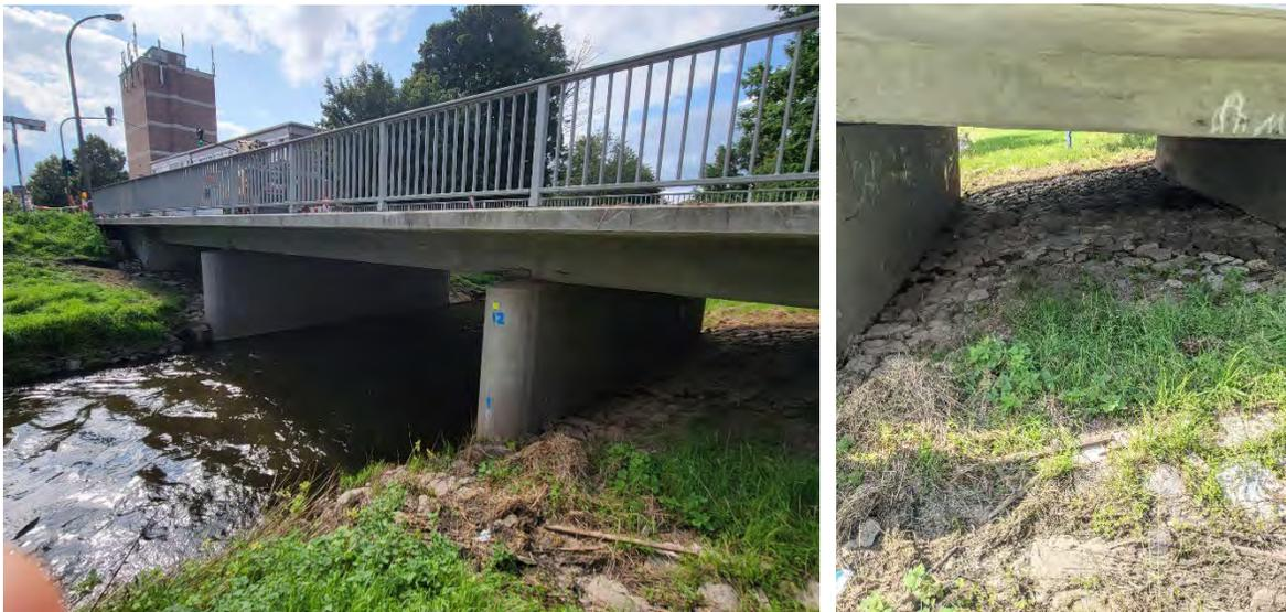
Figure 3.49. Photos of the Merowingerstrasse bridge across the Erft river in Bliesheim-Erfstadt. Left) Flowpaths and erosion was visible parallel to the bridge down the riverbank slopes. Right) Soil erosion on the riverbanks near the bridge abutments and piles and possibly removal of cobble slope reinforcement between the abutment and the pile are visible (50.782199; 6.822505)
