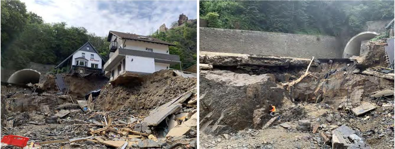
Figure 3.161. Left: extreme scour and erosion of the foundations of the residential buildings adjacent to the tunnel exit; right: washed out soil and rock just below the tunnel exit, causing a deep cut of 3+ meters, (50.5165261, 6.9975355)
