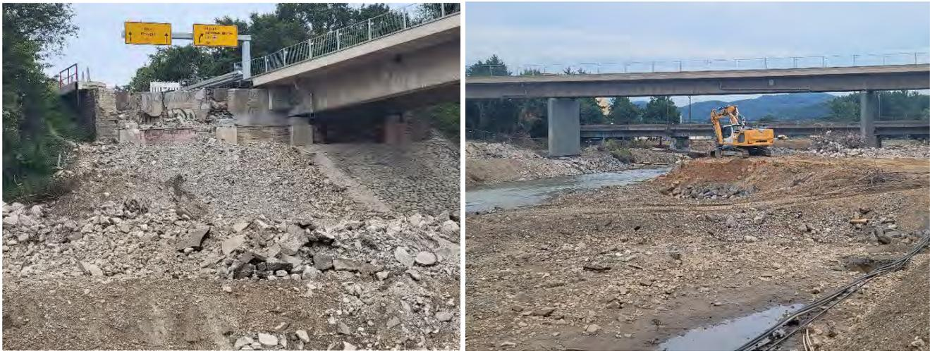
Figure 3.232. Left: Removed damaged bridge deck of the B9 in Sinzig on August 12, 2021, northern riverbank. Right: Active soil preparation and infill ongoing on the southern riverbank side (50.55218, 7.253561)
