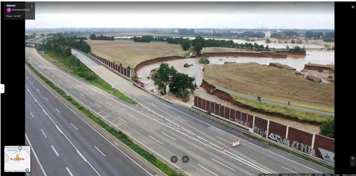
Figure 3.43. Aerial photograph showing damage to embankment and noise protection wall along freeway A1.
