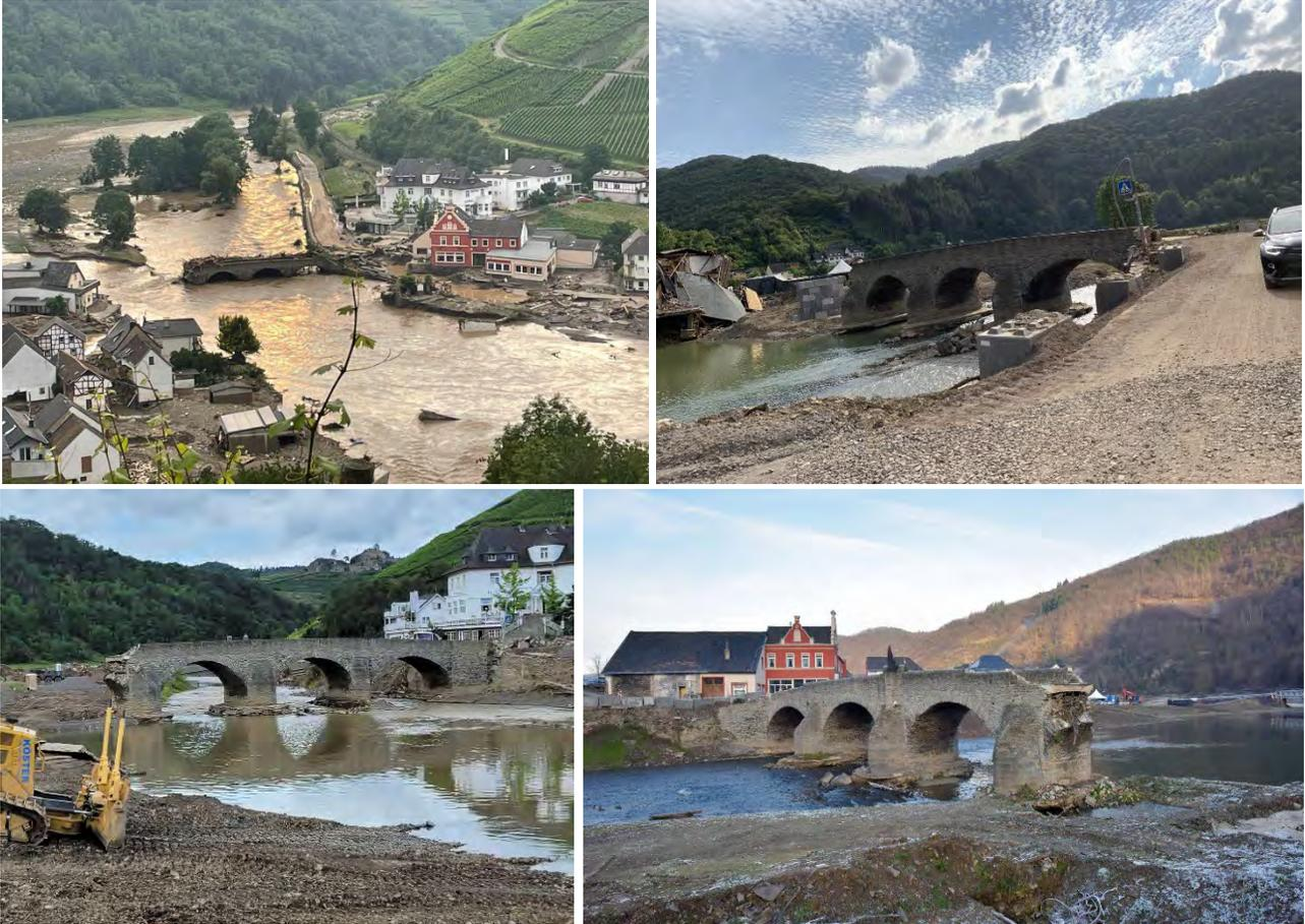
Figure 3.197. After flood photos of the Nepomuk bridge in Rech, showing missing bridge arch and abutment structure (50.5141233, 7.03625453)
