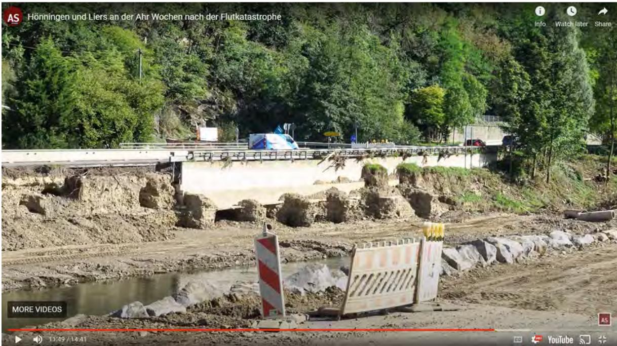
Figure 3.89. Embankment damage along road 273 in Hönningen, taken several weeks after the flood (source: Screenshot of video footage filmed by Alois Sheuer, source: <https://www.youtube.com/watch?v=6EXwo6ZxrFs> )
