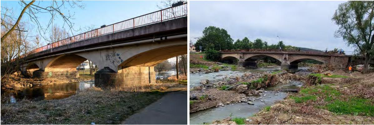
Figure 3.228. Koelner Strasse bridge crossing the Ahr in Sinzig (left, source: [https://www.aw-wiki.de/index.php/Ahrbr%C3%BCcken\\_im\\_Kreis\\_Ahrweiler](https://www.aw-wiki.de/index.php/Ahrbr%C3%BCcken_im_Kreis_Ahrweiler)) before the flood event and (right) at the time of the GEER-visit (August 12).
