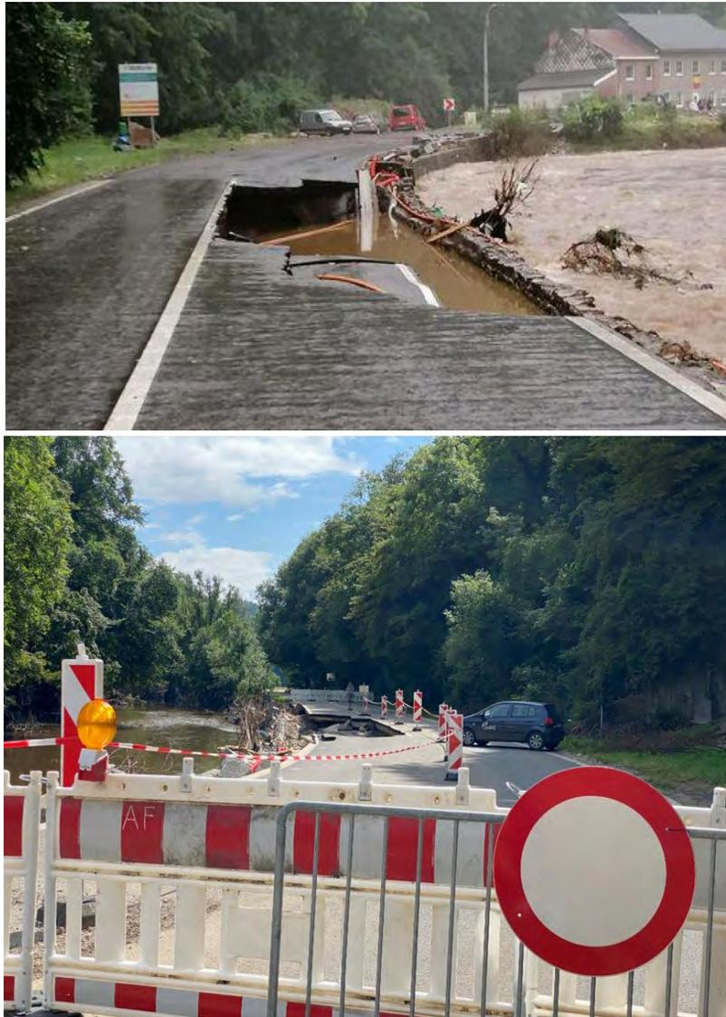
Figure 3.271. Road failure in N61 urban motorway between Dolhain and Verviers, along the river Vesdre. Top photograph source: <https://lameuse-verviers.sudinfo.be/814356/article/2021-08-01/la-n61-entre-dolhain-et-verviers-fermee-plusieurs-semaines-suite-aux-inondations>. Bottom Photograph source: [https://www.lavenir.net/cnt/dmf20210731\\_01601829/la-nationale-entre-dolhain-et-verviers-est-fermee](https://www.lavenir.net/cnt/dmf20210731_01601829/la-nationale-entre-dolhain-et-verviers-est-fermee)
