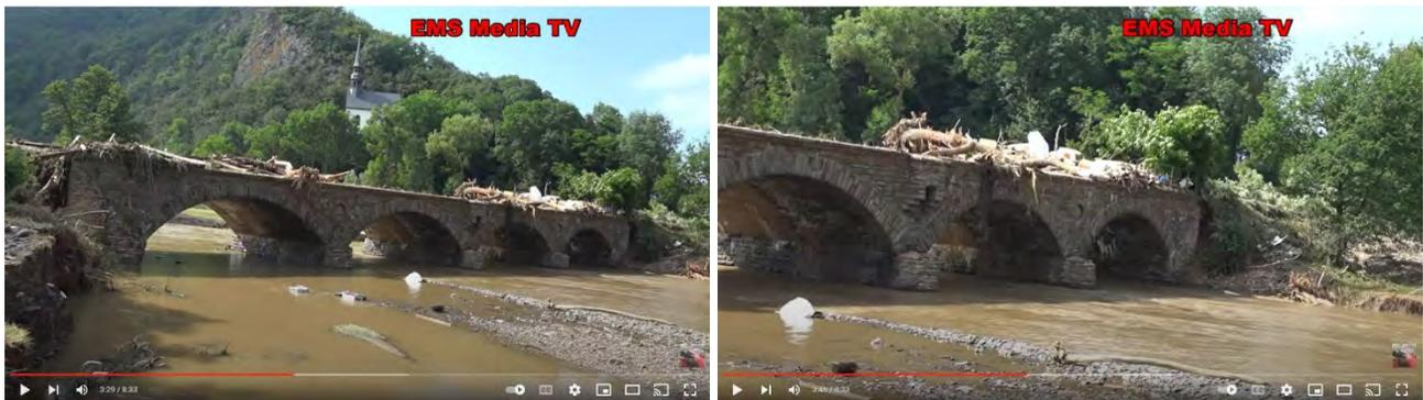
Figure 3.115. Railroad bridge from downstream direction shortly after the flood showing massive amounts of debris and deadwood piled up around bridge structure, Source: <https://www.youtube.com/watch?v=MSrJRXI6dQA>
