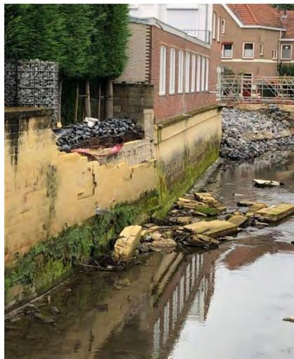
Figure 3.280. Retaining wall failure along the Geul river in Valkenburg ( $50^{\circ}51'54.3''N$   $5^{\circ}49'49.8''E$ )
