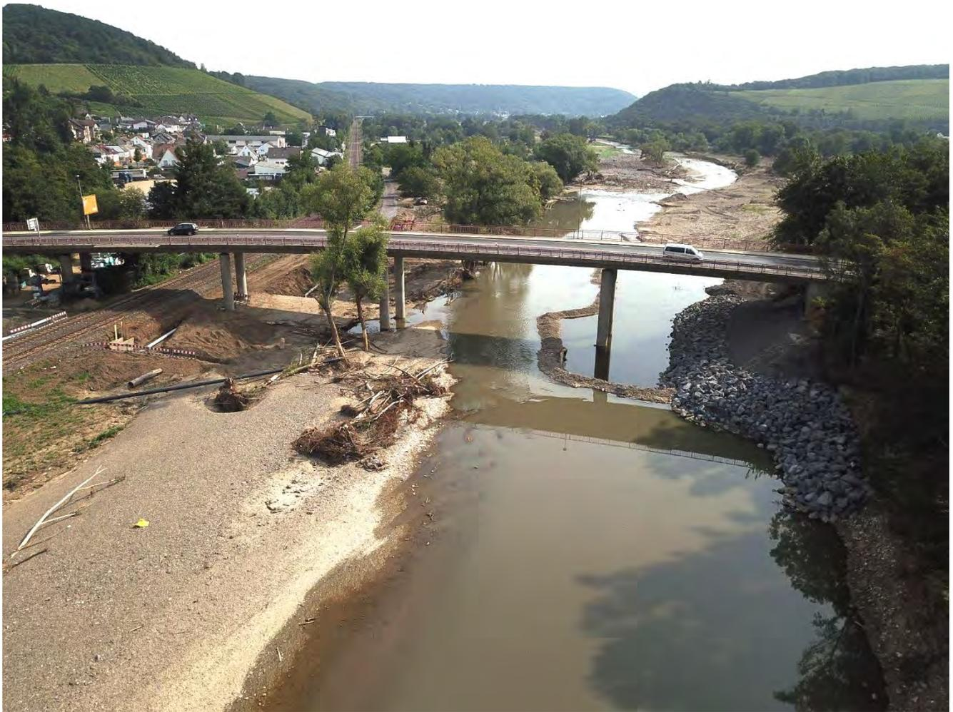
*Figure 3.227. Recent gravel and riprap deposits supporting the bridge abutments in Green (50.5470057, 7.18318548).*
