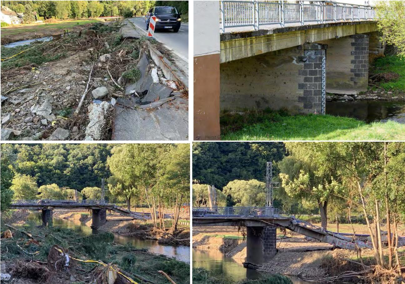
Figure 3.57. Road and Bridge damage in Müsch. Top left: Road damage along the L73, Top right: Bridge prior to flood, Bottom left: damaged bridge in August 2021, Bottom right: close up of missing abutment and collapse of bridge deck (50.385952, 6.8288141)
