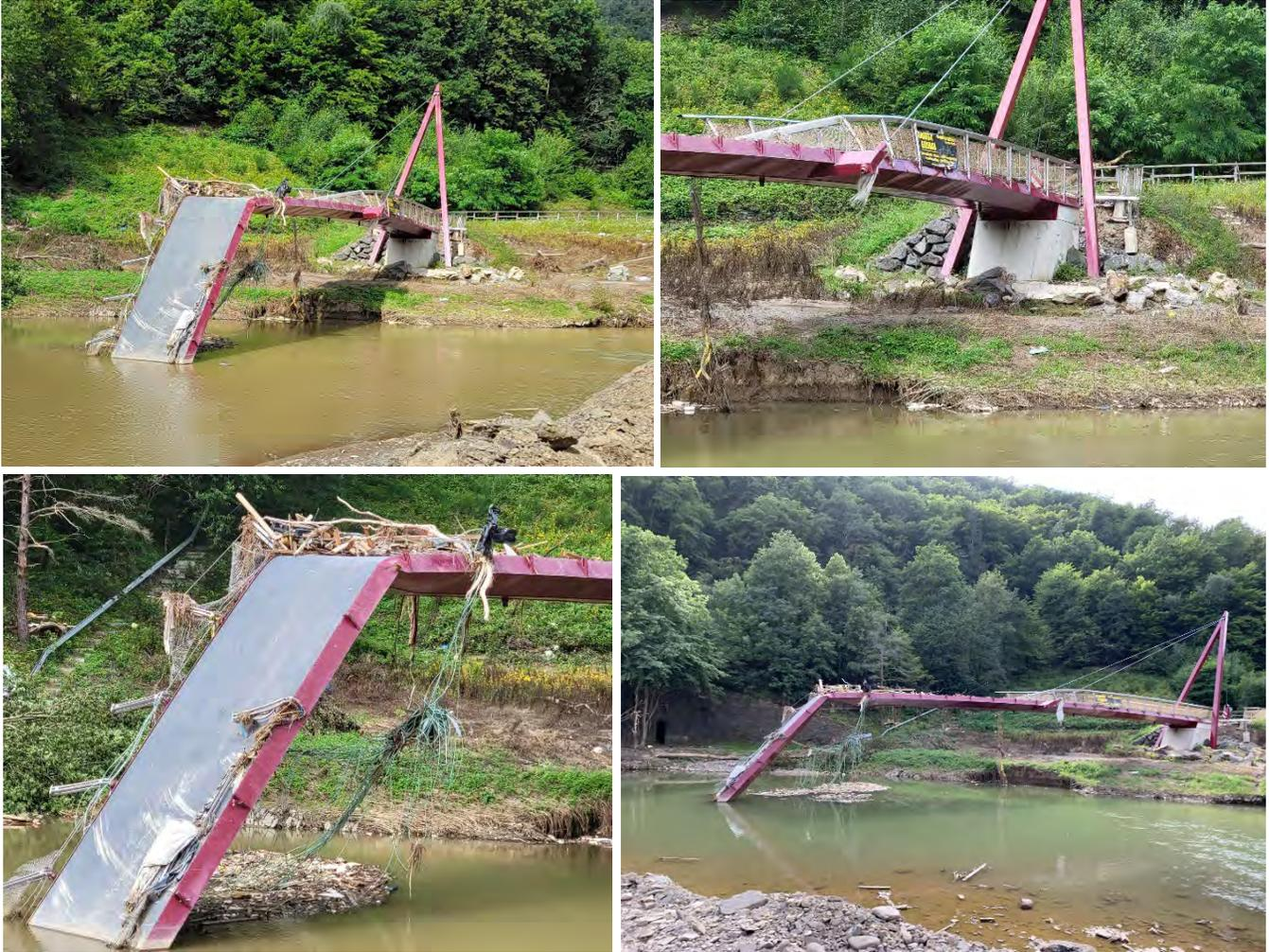
Figure 3.174. Bridge damage of the bicycle bridge in Reimerzhoven documented by the GEER team (50.5188435, 7.00714039)
