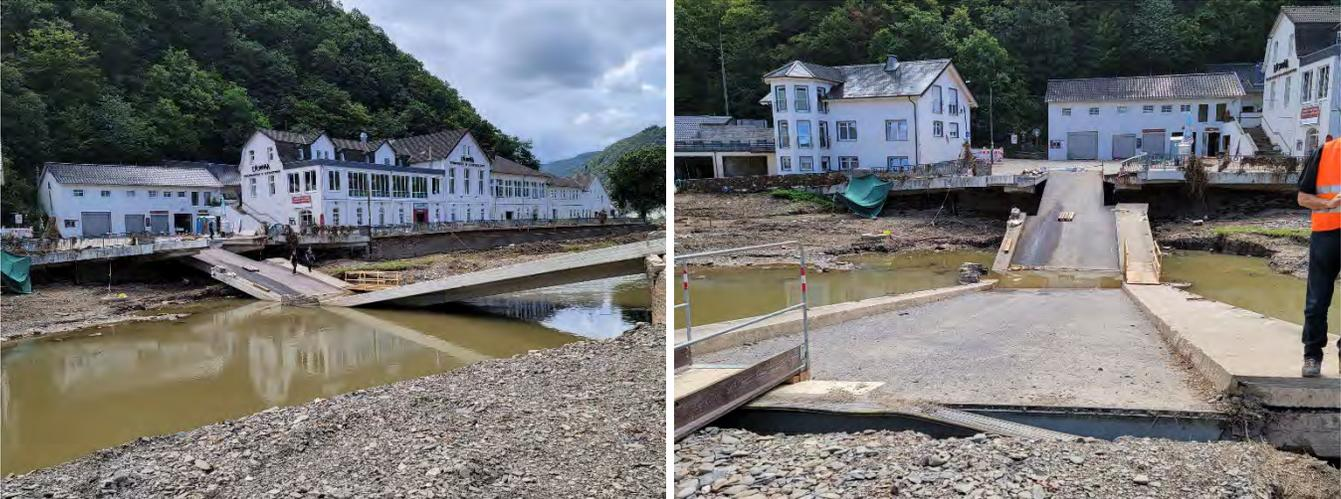
Figure 3.201. Damaged Ahr bridge in Dernau on August 10th, 2021, documented by the GEER team (50.533719356, 7.0453862)
