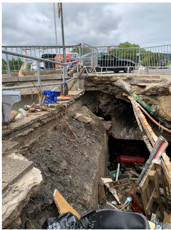
Figure 3.244. Pont du L'honneux damage: left embankment wall in upstream direction(50.609966, 5.6194468).
