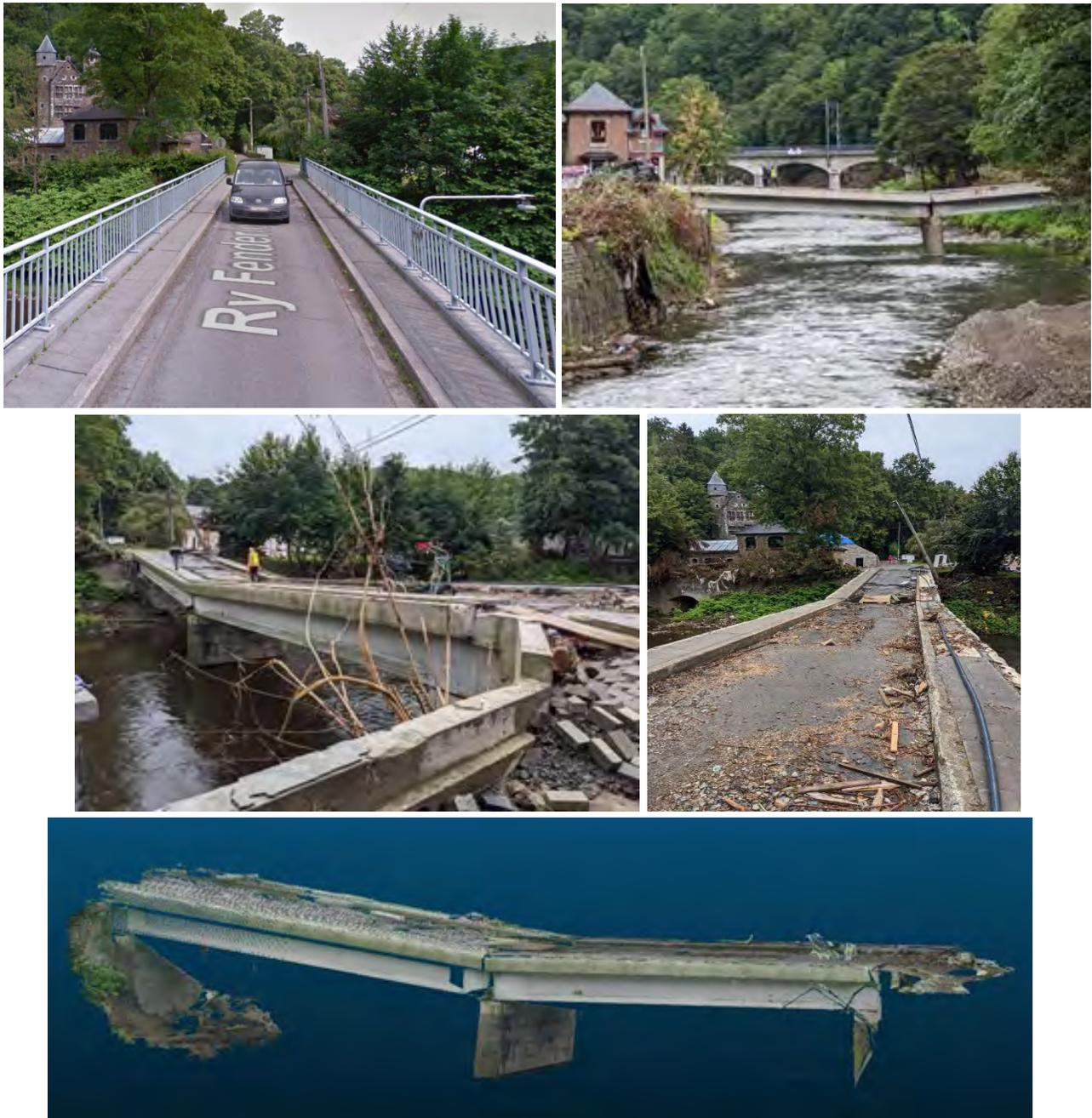
Figure 3.259. Photographs and point cloud model (13.5 million points) obtained from LiDAR scanning (Location: Trooz, Belgium 50.571160, 5.689884, Rue de Verviers 6, 4870 Trooz & Ry Fenderie)
