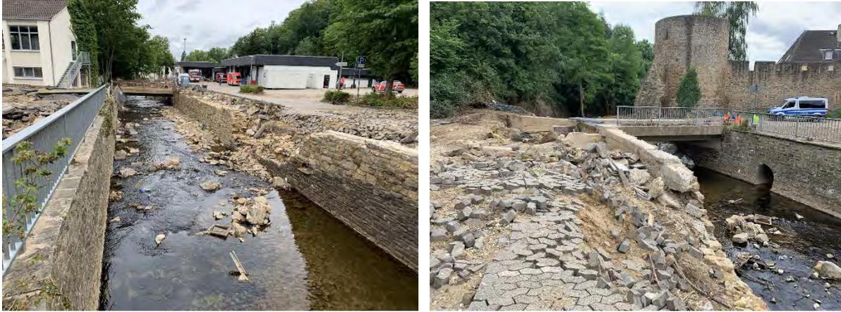
Figure 3.12. Embankment damage just below the bridge structure (50.55748613, 6.7659919).
