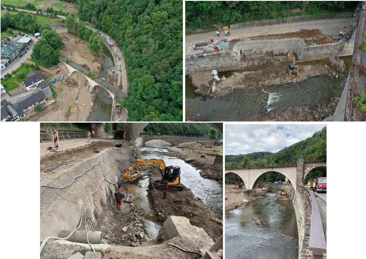
Figure 3.58. Localized Embankment failure in Fuchshofen and ongoing repair work (50.429957, 6.850187)
