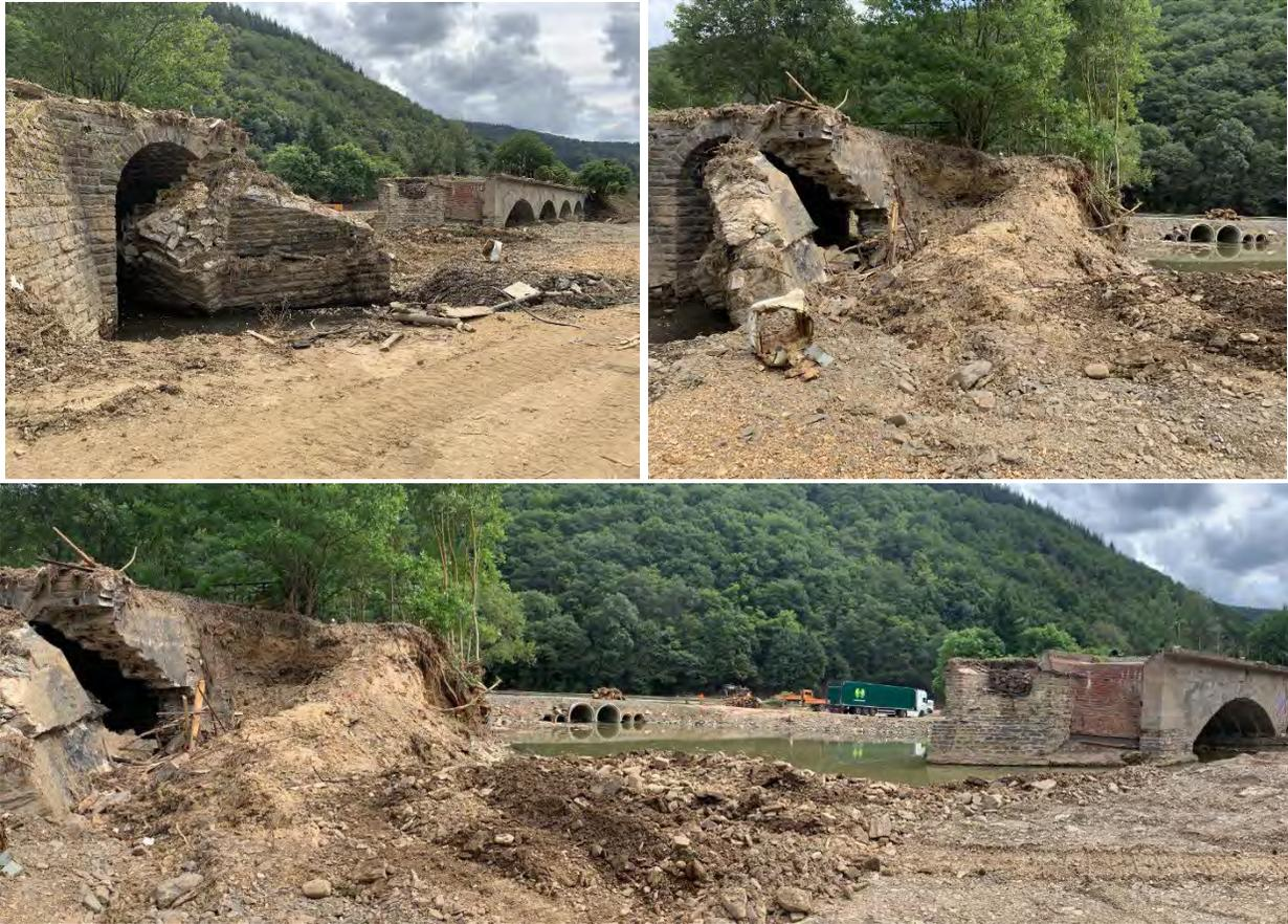
Figure 3.98. Photo of damaged bicycle tunnel from upstream direction showing washed out soil (dam) segment in between the two structures and the temporary water rerouting (pipes) in the background (50.480833, 6.968818).
