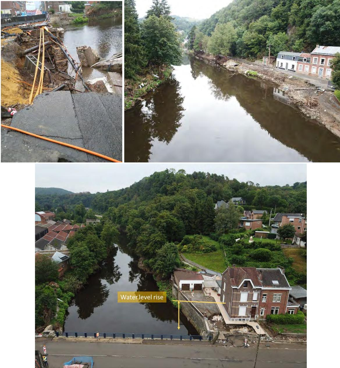
Figure 3.258. Damage of abutment and wingwall area on the other side of the road bridge, (50.574176, 5.742544).
