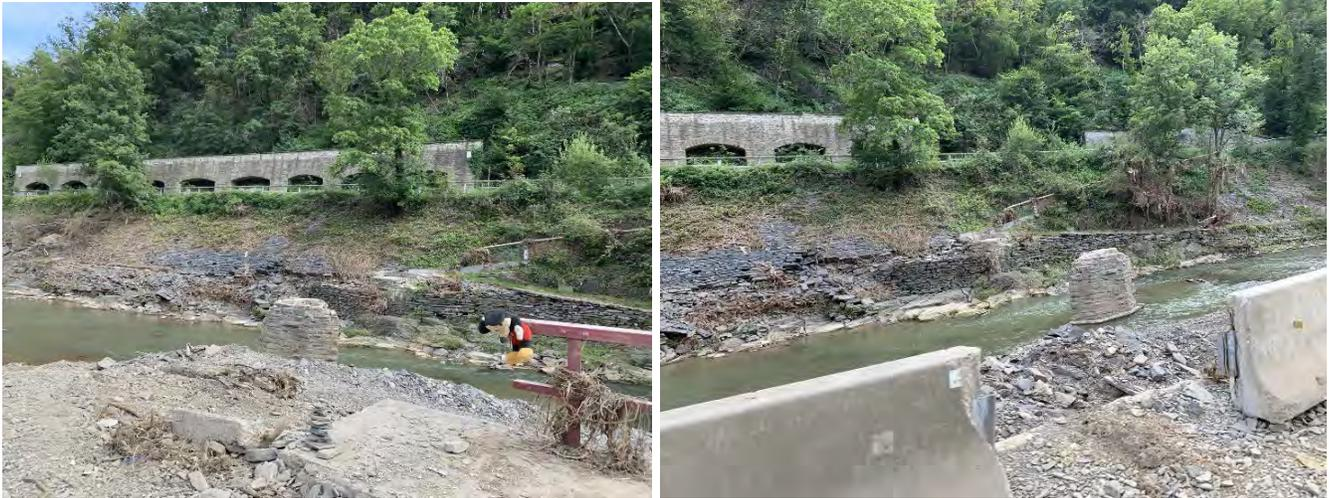
Figure 3.170. Remaining middle pier of pedestrian bridge in Reimerzhoven, and soil erosion near embankment (50.5195072, 7.004132)
