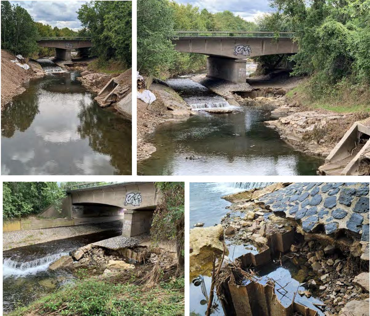
Figure 3.20. Foundation damage at middle pier of railway bridge (50.660347, 6.805227)
