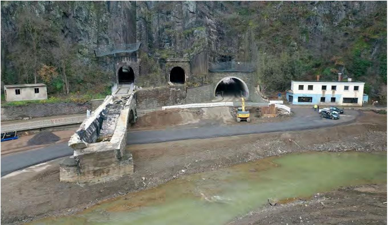
*Figure 3.152. Tunnel Entrance, October 2021. Only one bridge arch remains, reconstruction of road access, one bridge was completely demolished. Source: unknown, GPS Coordinates: 50.51637961742962, 6.995167798855734.*
