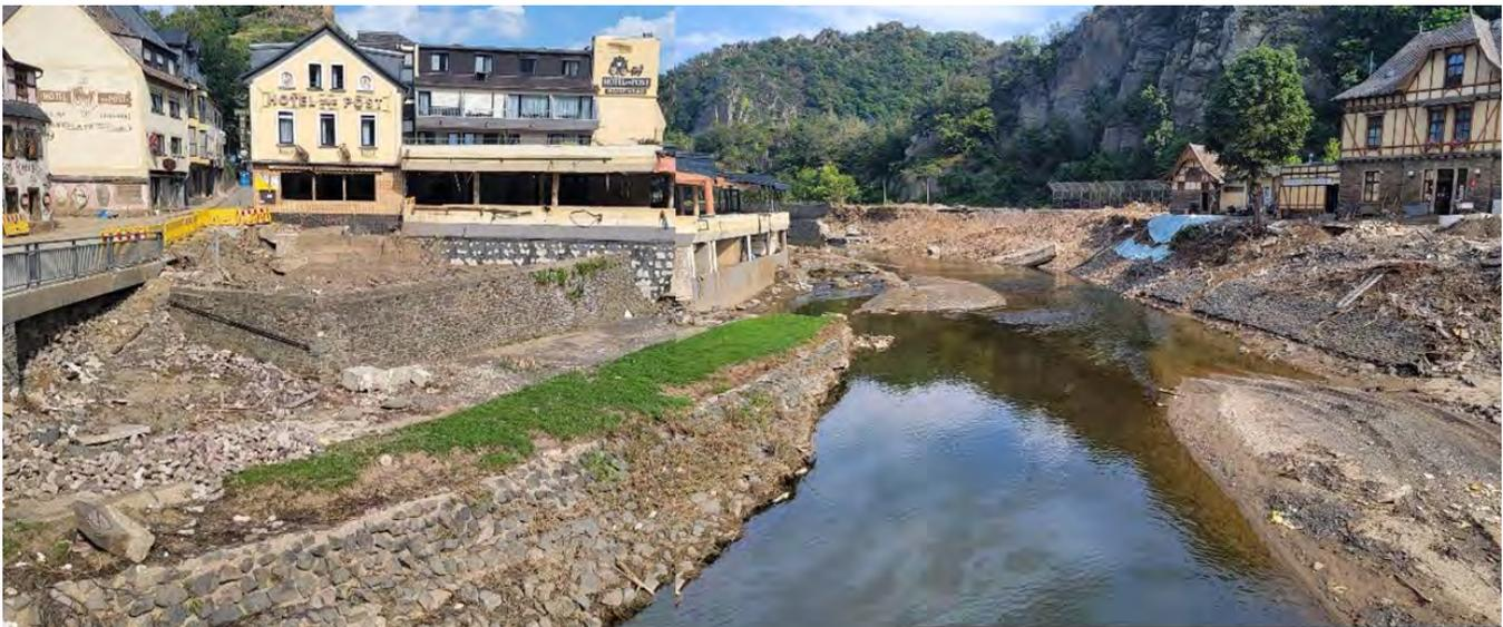
Figure 3.143. Photograph taken from the road bridge in the town center looking at the Ahr and the adjacent "Hotel zur Post"; embankment damage on both sides; Train station to the right (50.5165073, 6.98911282)
