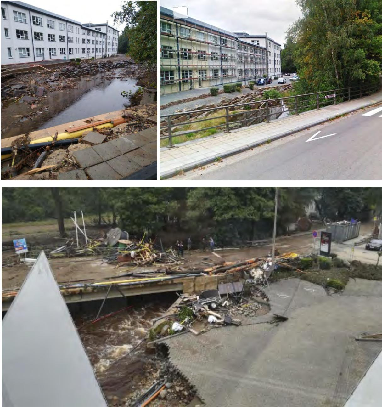
Figure 3.273. Top: Gravity wall failure in Eupen (exact location: 50.614888, 6.045164), Bottom: Parking lot collapse due to river bank being washed out and traffic interrupted. Main entrance of the Arbeitsamt der Deutschsprachigen Gemeinschaft Belgiens, Eupen in Belgium. Source: <https://www.grenzecho.net/59306/artikel/2021-07-21/arbeitsamt-der-dg-zieht-vorubergehend-die-oberstadt>
