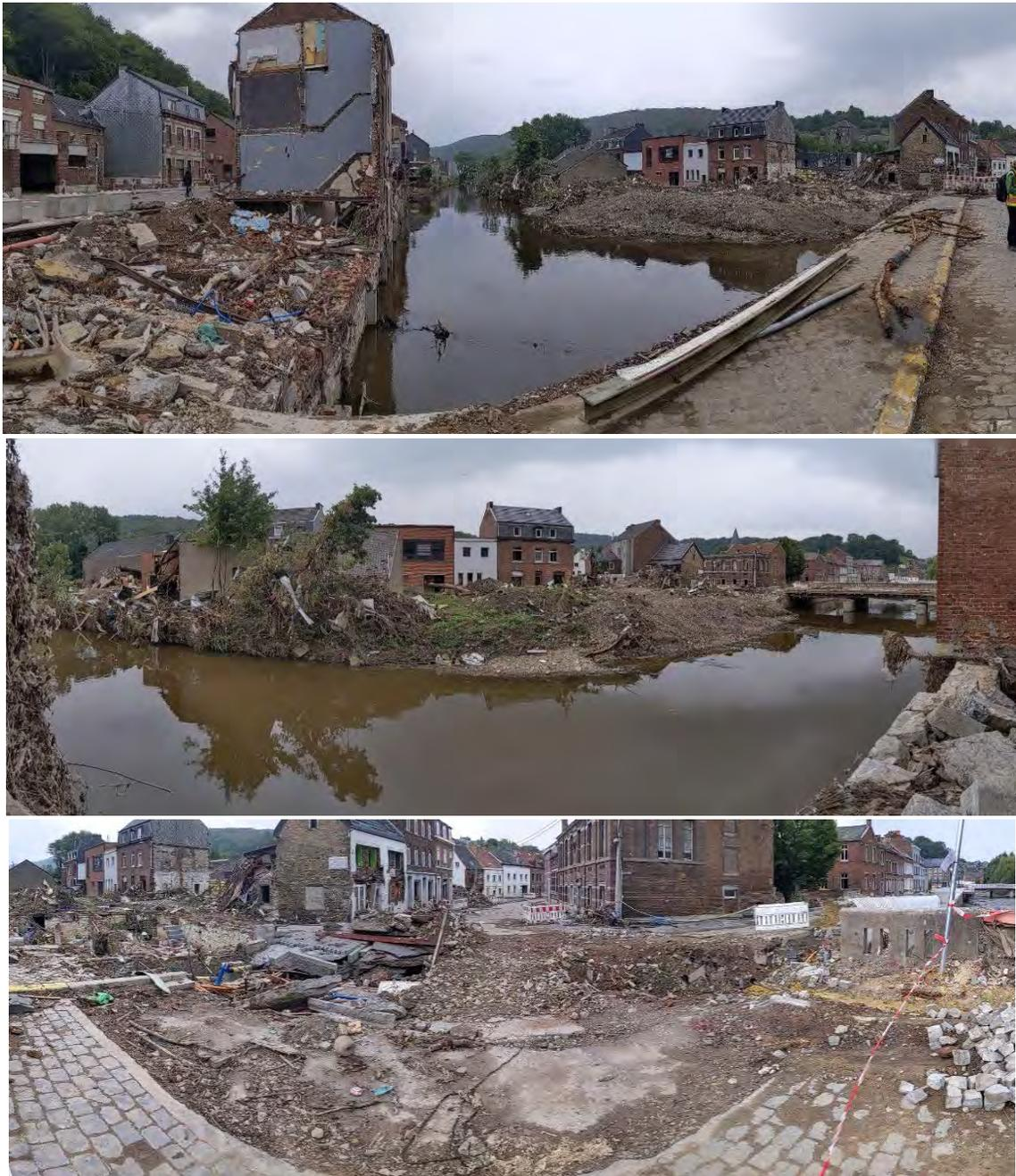
Figure 3.267. Photographs of flood damage in Pepinster (top: residential destruction, middle: embankment failure, bottom: road and foundation failures), (50.569710, 5.804977).
