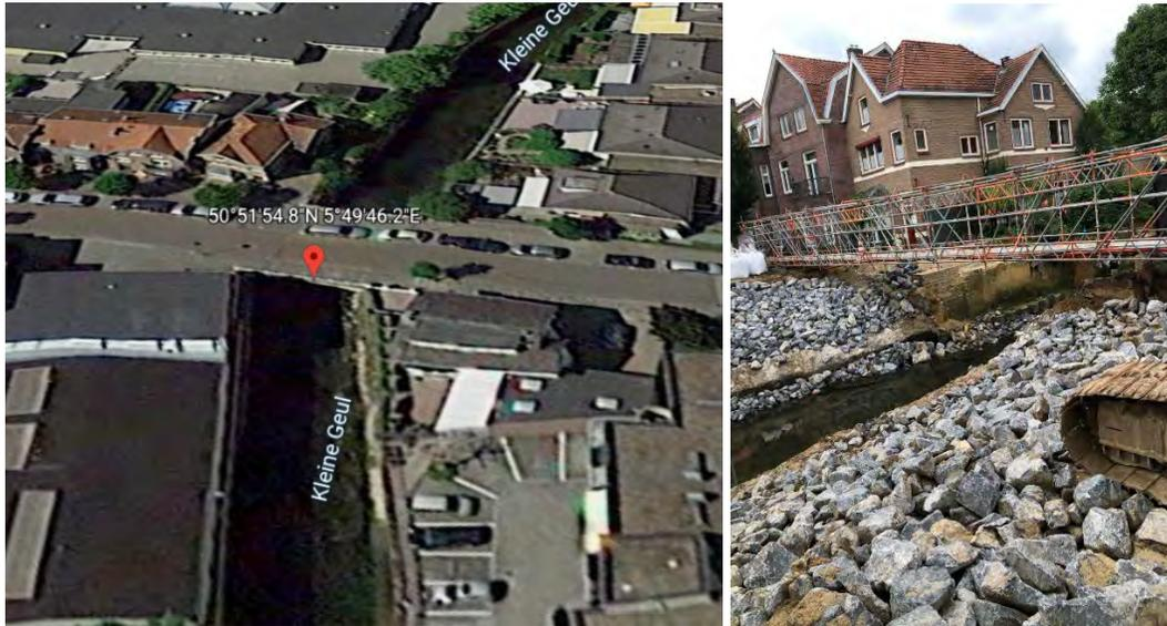
Figure 3.281. Temporary pedestrian bridge in place of a destroyed two-lane bridge (50°51'54.8"N 5°49'46.2"E)
