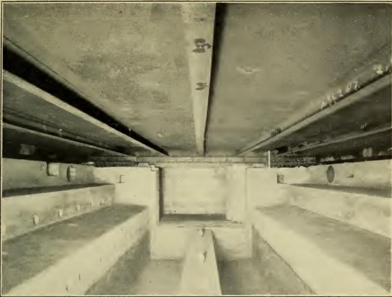
FIGURE 4.—Lower surface of the completed floor ready for test.
