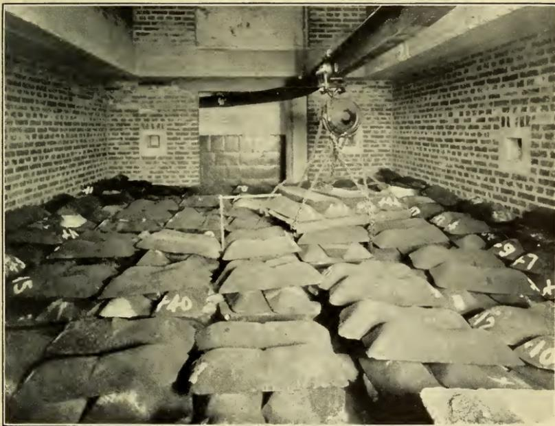
FIGURE 5.—The floor under a nominal load of 420 pounds per square foot of loaded area.
